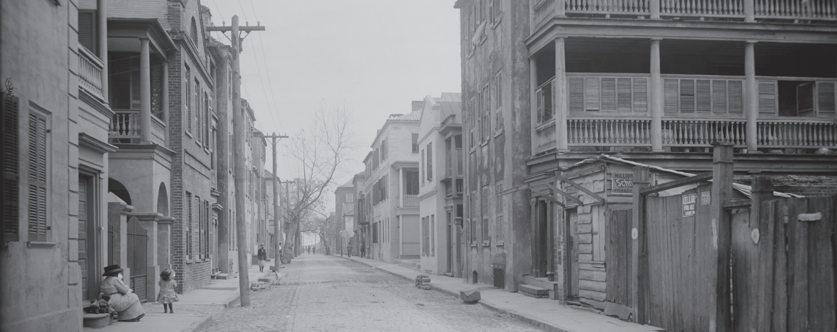
Charleston's early architecture relied on windows and piazzas for natural ventilation and shade. (www.loc.gov)
