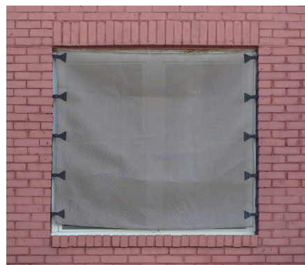
Fabric panels are an option for temporary protection that can be easily stored and installed prior to a storm.
