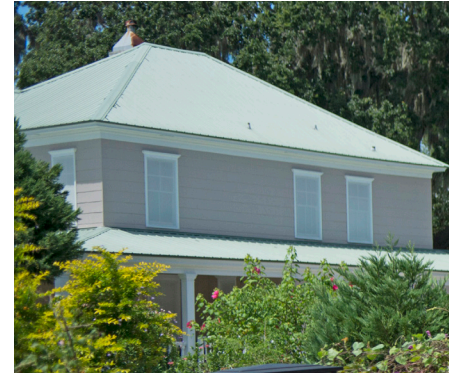
Shade shutters are used during the day to block strong sun exposure.
