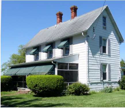
Historic porches, awnings, and traditional shutters shield building walls and openings from the sun.
