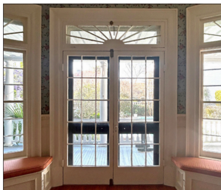
French doors can have upper and lower lock mechanisms to help secure them in place during strong winds.
