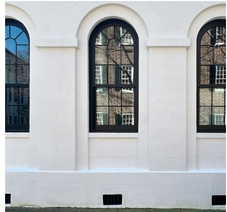
Window openings can be altered while still revealing the architectural character of the molding details.
