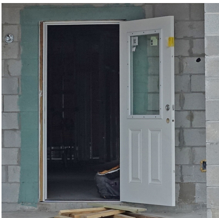
Composite doors are made of multiple layers of different materials, often with a steel or fiberglass finish.
