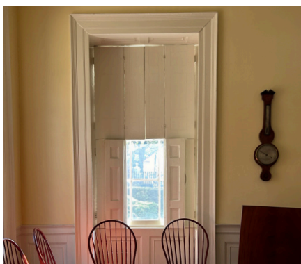
Shutters may also be used on the interior to limit sunlight and act as a secondary barrier protection.
