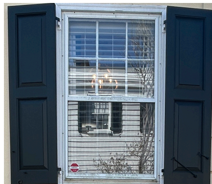
Storm windows with tempered glass or impact-resistant glazing provide protection from windborne debris. (Not approved on historic properties.)
