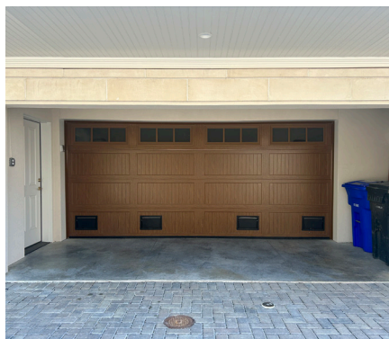
Garage doors are available with flood vents and structural ratings to resist flood and wind pressure. (Refer to Garage Door Wind Protection , sidebar page R6.9.)
