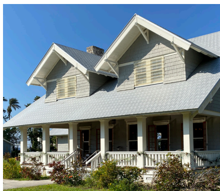
Polycarbonate shutters allow light to enter a building but are used for temporary purposes in the event of a storm.
