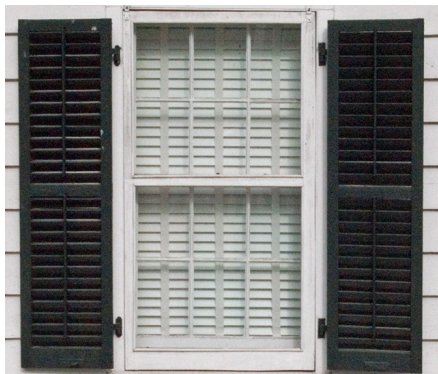
Traditional wood shutters are designed to close and fully cover window openings, and can provide some protection from airborne debris.
