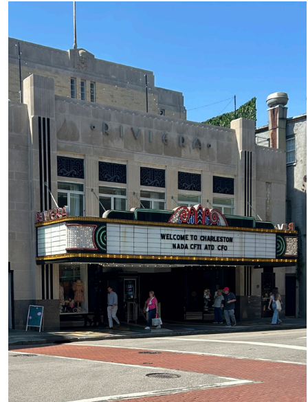
Many older buildings use unreinforced masonry construction, which is more vulnerable to seismic events.
