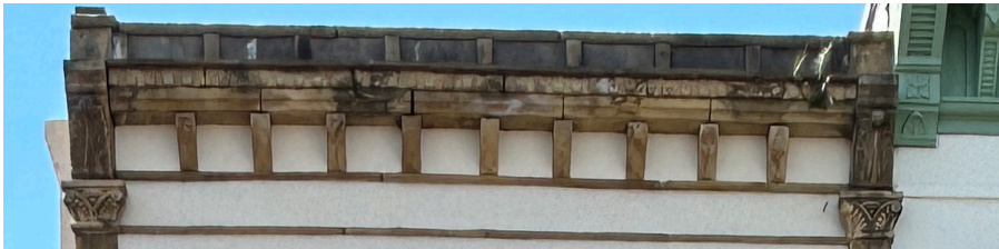
Terra cotta is made of clay, cast in molds similar to brick, in a variety of decorative shapes and colors. Decorative terra cotta is usually non-structural.
