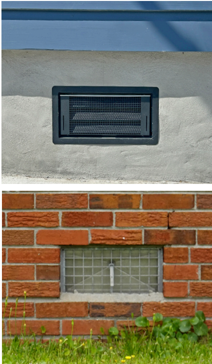
Flood vents may be installed new, or in existing openings in a foundation if they meet design and spacing requirements.
