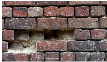
Deteriorated surfaces and mortar are more likely to absorb moisture.
