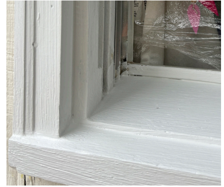
After painting, the repaired area is difficult to distinguish from the wood.
