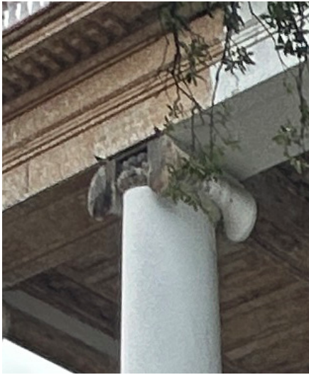
Trim pieces may appear as monolithic, solid features, however they are usually made up of many pieces.
