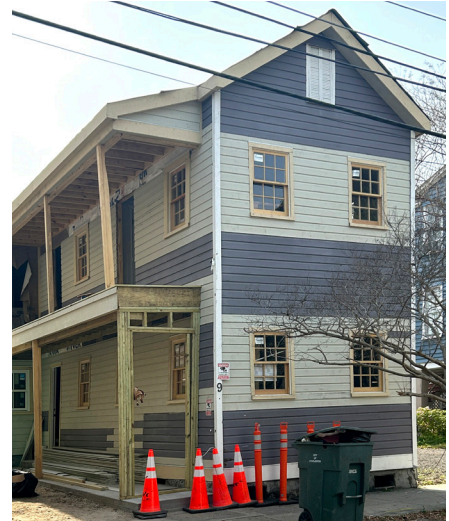
Removal of original siding should be limited because old-growth wood is dense and more decay resistant.
