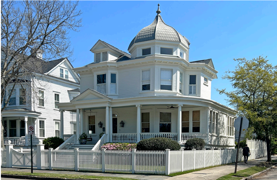
All wood surface elements and details should be securely fastened, regularly repainted, and monitored for rot to increase resistance to natural hazards.
