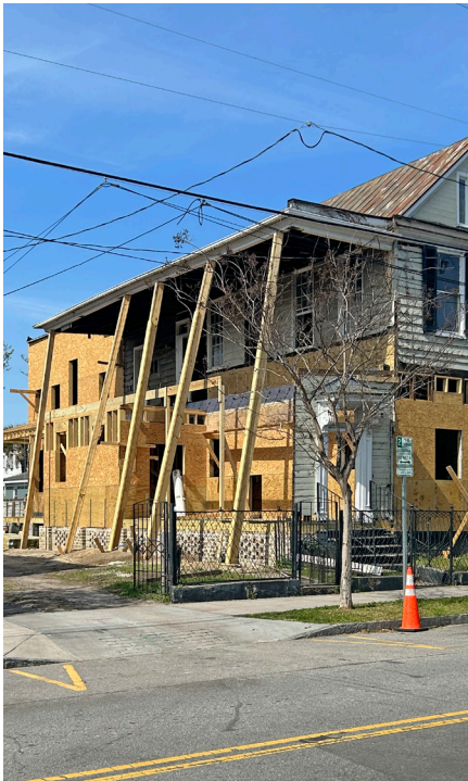
Shear panels can be installed on outside walls when siding is being replaced.
