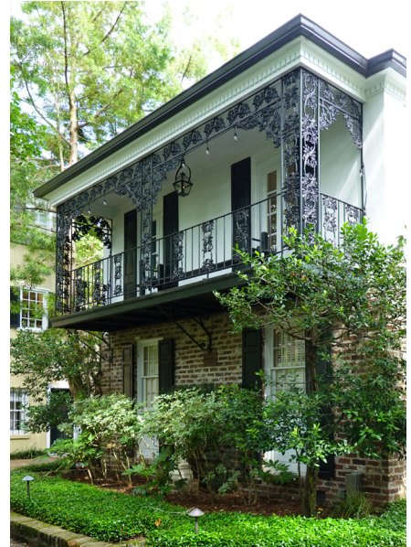
A few buildings in the historic district feature wrought or cast iron detailing in balconies or galleries, that should be retained and preserved to the extent possible. (Refer to NPS Preservation Brief 27: The Maintenance and Repair of Architectural Cast Iron for additional resources.)
