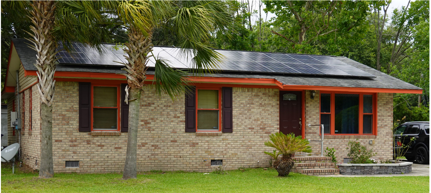
The visibility of solar panels can be reduced if the color is close to the roof surface color. Verify that attachments are appropriate for the roof materials and securely fastened to reduce the likelihood of uplift in severe winds.
