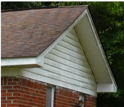
Overhangs on most buildings extend up to 16-inches from the building wall.
