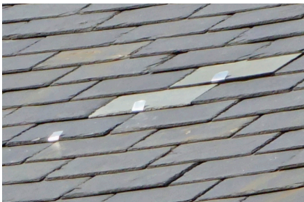
Metal hangers can be used to secure dislodged slates or replace individual slates.
