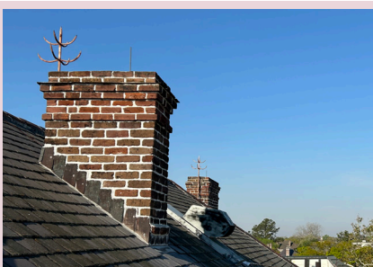
Lightning rods look like spikes sticking up from the roof surface.
