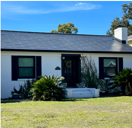
Solar roof tiles can more closely mimic shingle patterns.
