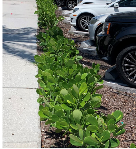
Portions of this parking lot have been curbed to allow for planting areas that increase the capacity for stormwater.
