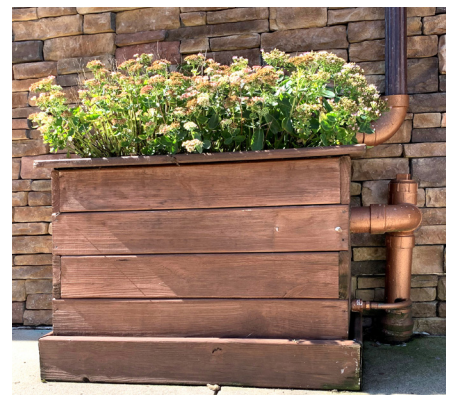
Hybrid rain barrels can capture stormwater and support plantings or small gardens in paved area.
