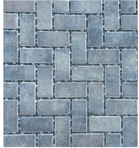
Pavers are available with edge spacers that form open, pervious joints when laid, allowing water to flow through into the ground.
