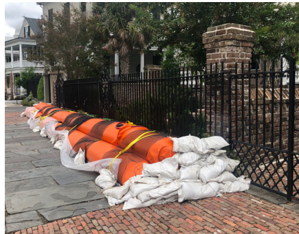
Temporary barriers can reduce flood risk for a short duration if installed prior to an event. (Courtesy of Glenn Keyes)
