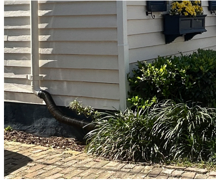
A solid downspout drain can divert water to a an absorption area or rain barrel.
