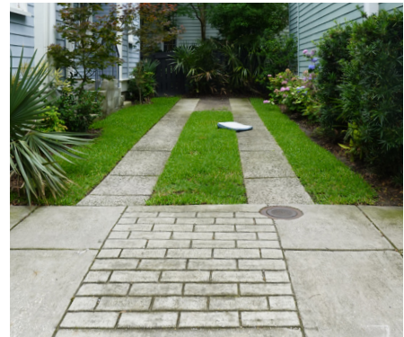
Driveways can be limited to tire paths or paved with pervious materials to increase the ability for stormwater to be captured on site.
