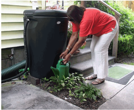
Rain barrels can be used as an irrigation source. (NC Cooperative Extension, www.ces.ncu.edu )
