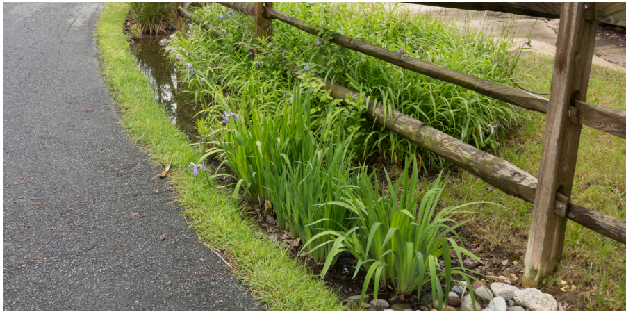
Rain gardens located along paved areas can collect roadway stormwater.
