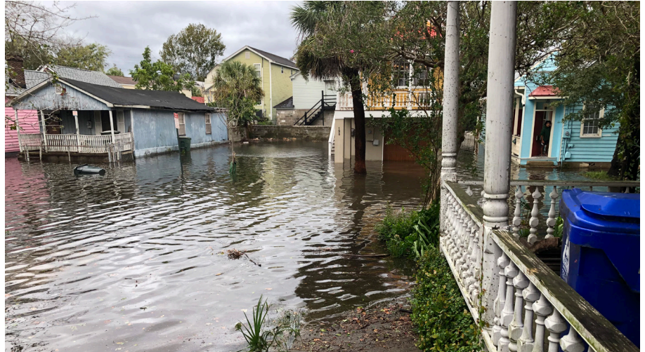
Flooding in the West Side. (Photo from PSC Survey, Brandon Hall)
