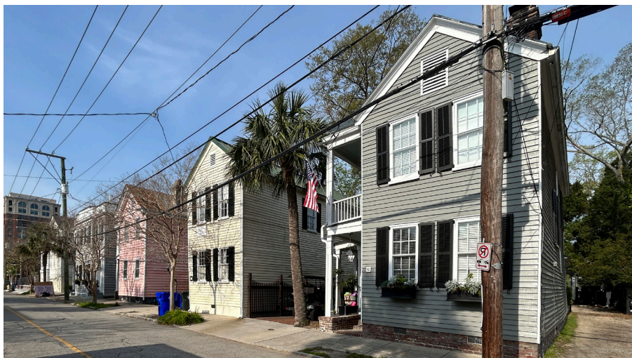
The southern exposures of several houses around 5pm see little relief from natural landscaping. Interior blinds can help reduce thermal energy radiating through the windows.
