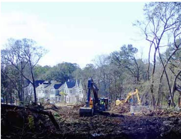
Site preparation removes the forest, topsoil, and roots leaving only grand trees that are protected by law.
