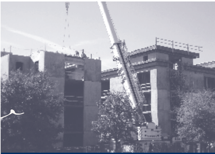
Standard Precut Walls are designed to withstand 180mph winds. Additionally, they stand up against some of the lowcountry's most fierce maintenance problems such as mold, insects, rot and fire.
