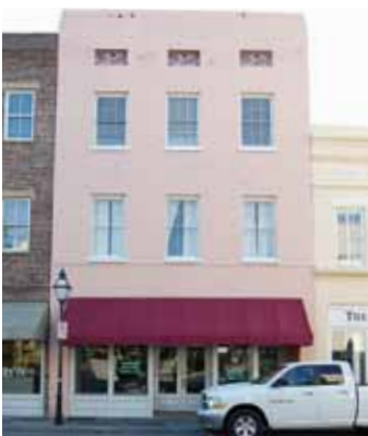
CAROLOPOLIS AWARD 169 King Street JOSEPH BALLARD BUILDING
