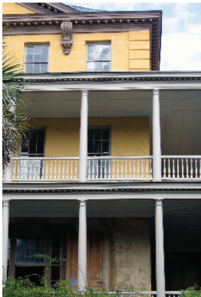
The completed top floor includes light scoring to simulate mortar between faux stone blocks. Second floor work (in progress) shows marked color contrast to the first floor as yet unrestored.
