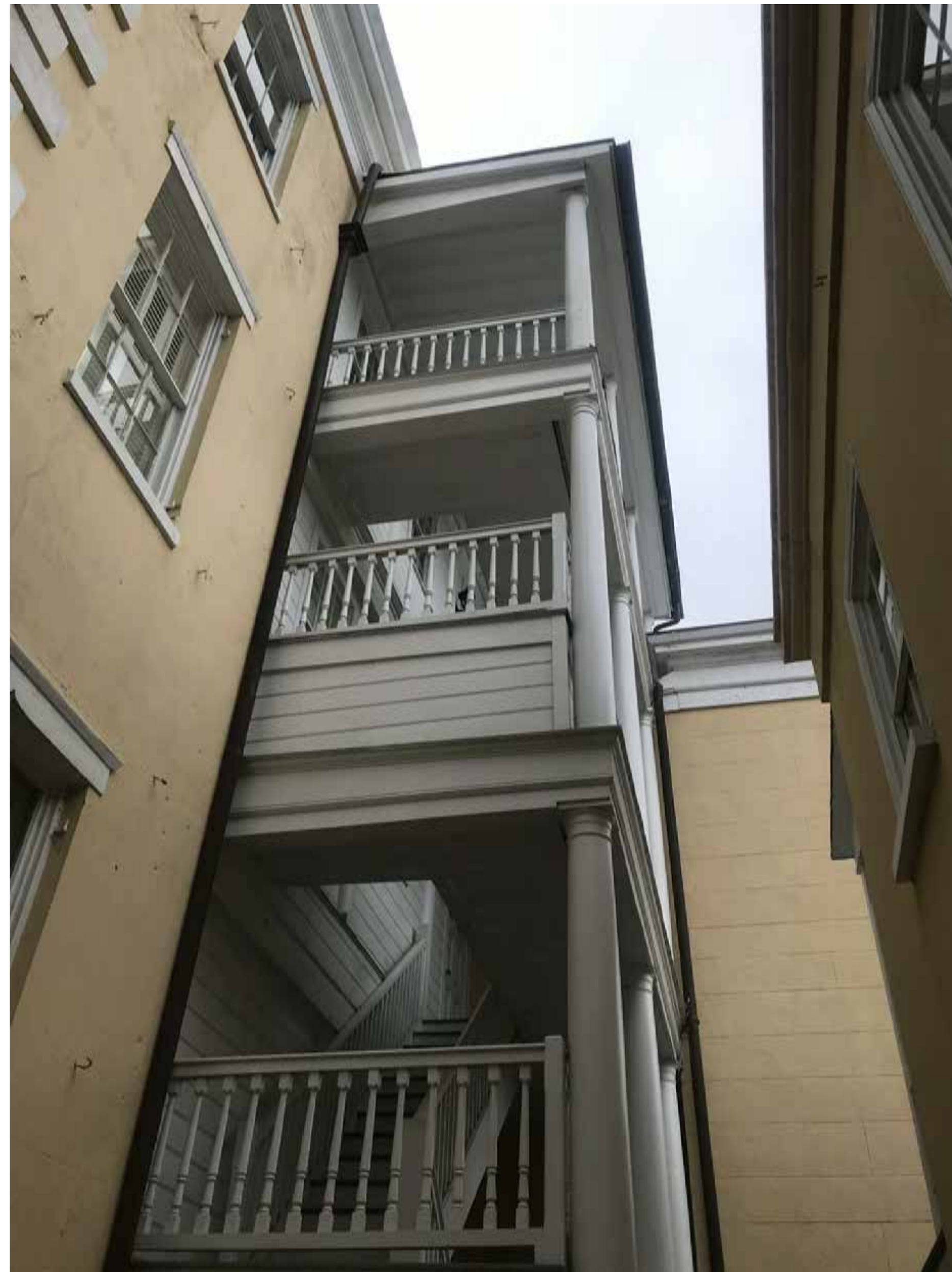
PHOTO 11: EXISTING VIEW OF PORCH AT REAR FROM CARRIAGE HOUSE
