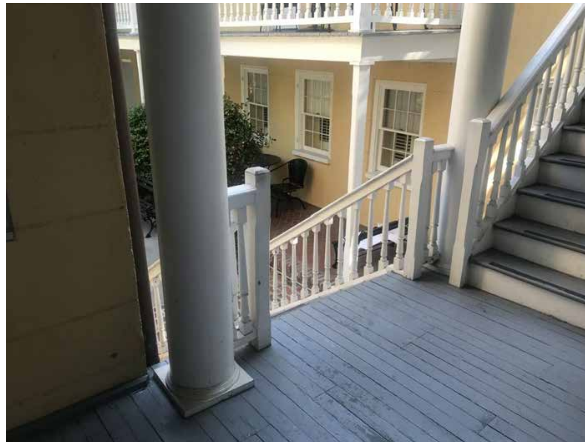
PHOTO 8: EXISTING VIEW OF STAIRS FROM FIRST FLOOR PORCH
