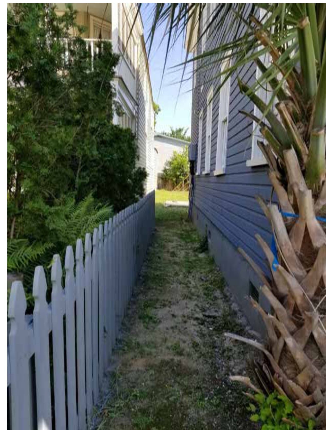
VIEW OF WEST SIDE ELEVATION FROM JUDITH STREET
