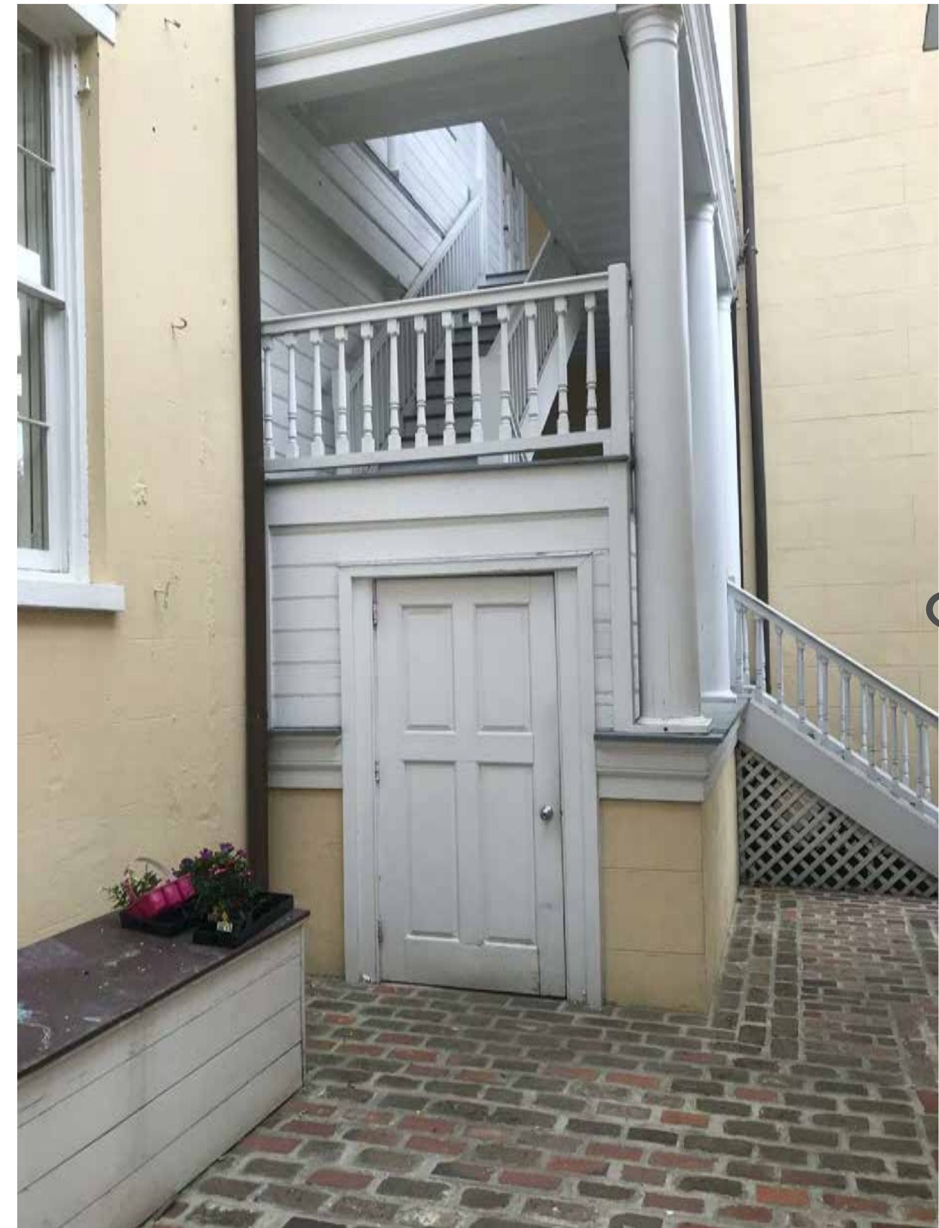
PHOTO 12 - EXISTING VIEW OF PORCH AT REAR FROM CARRIAGE HOUSE
