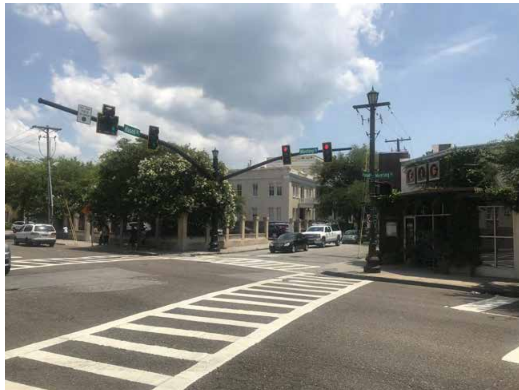
PHOTO 1: EXISTING VIEW OF PARAPET FROM CORNER OF MEETING HASALL STREETS (WEST ELEVATION)
