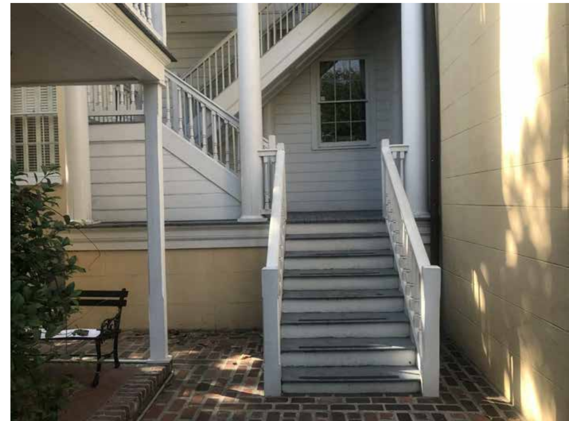
PHOTO 9: EXISTING VIEW OF PORCH/STAIRS FROM REAR PATIO
