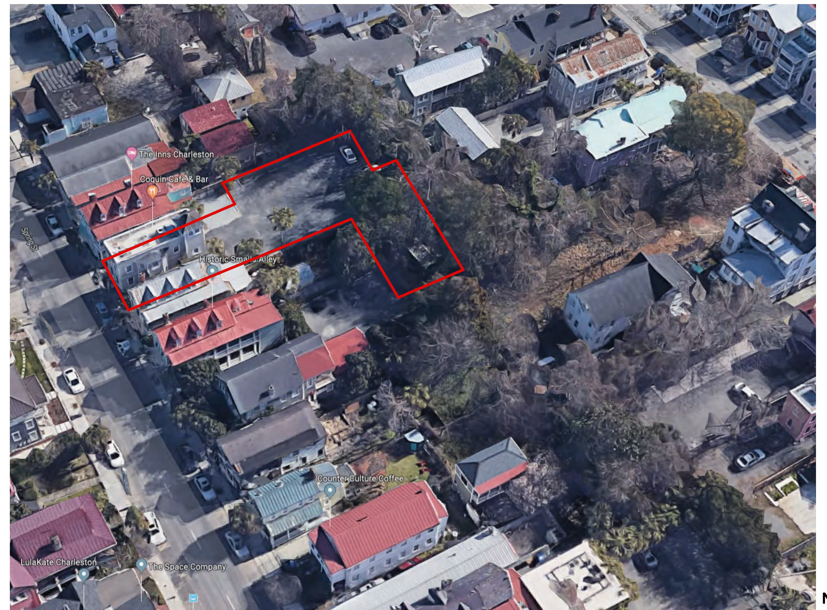
AERIAL VIEW: looking east
