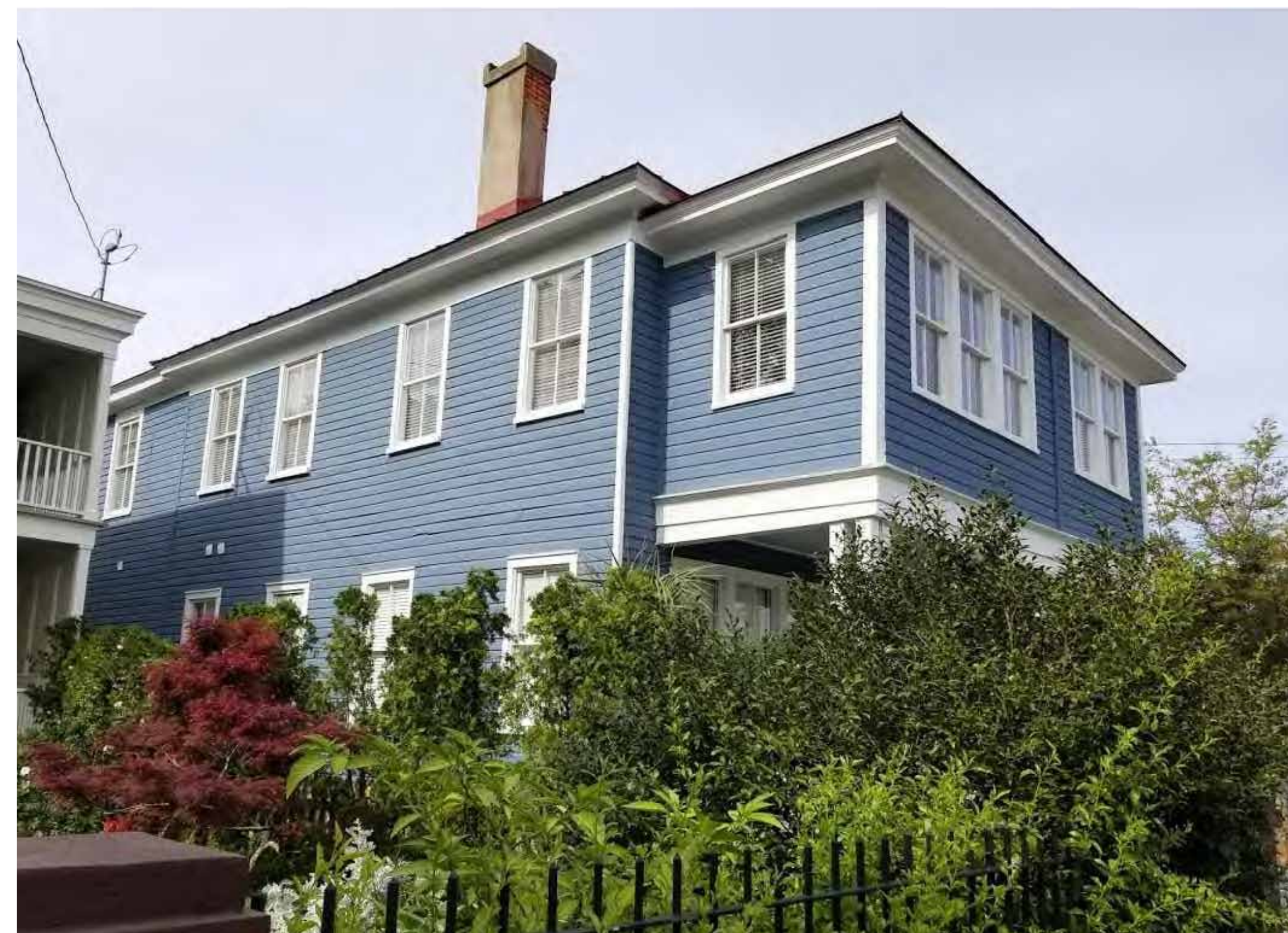
VIEW OF WEST ELEVATION FROM JUDITH
