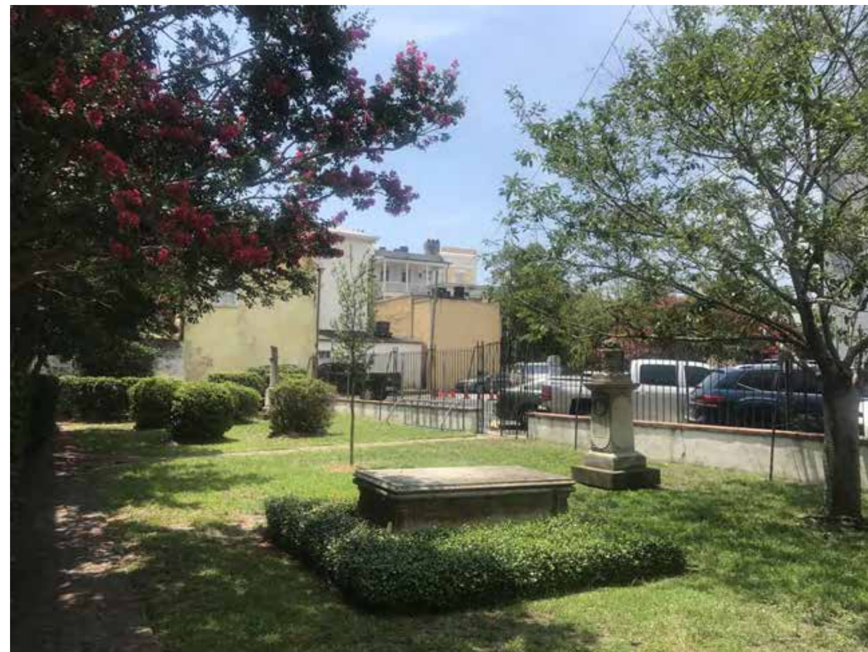
PHOTO 2: EXISTING VIEW OF HOUSE/PORCH FROM WENTWORTH STREET (NORTH ELEVATION)
