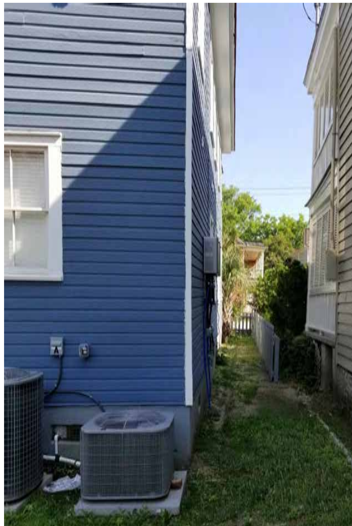
VIEW OF NORTH WEST CORNER ELEVATION
