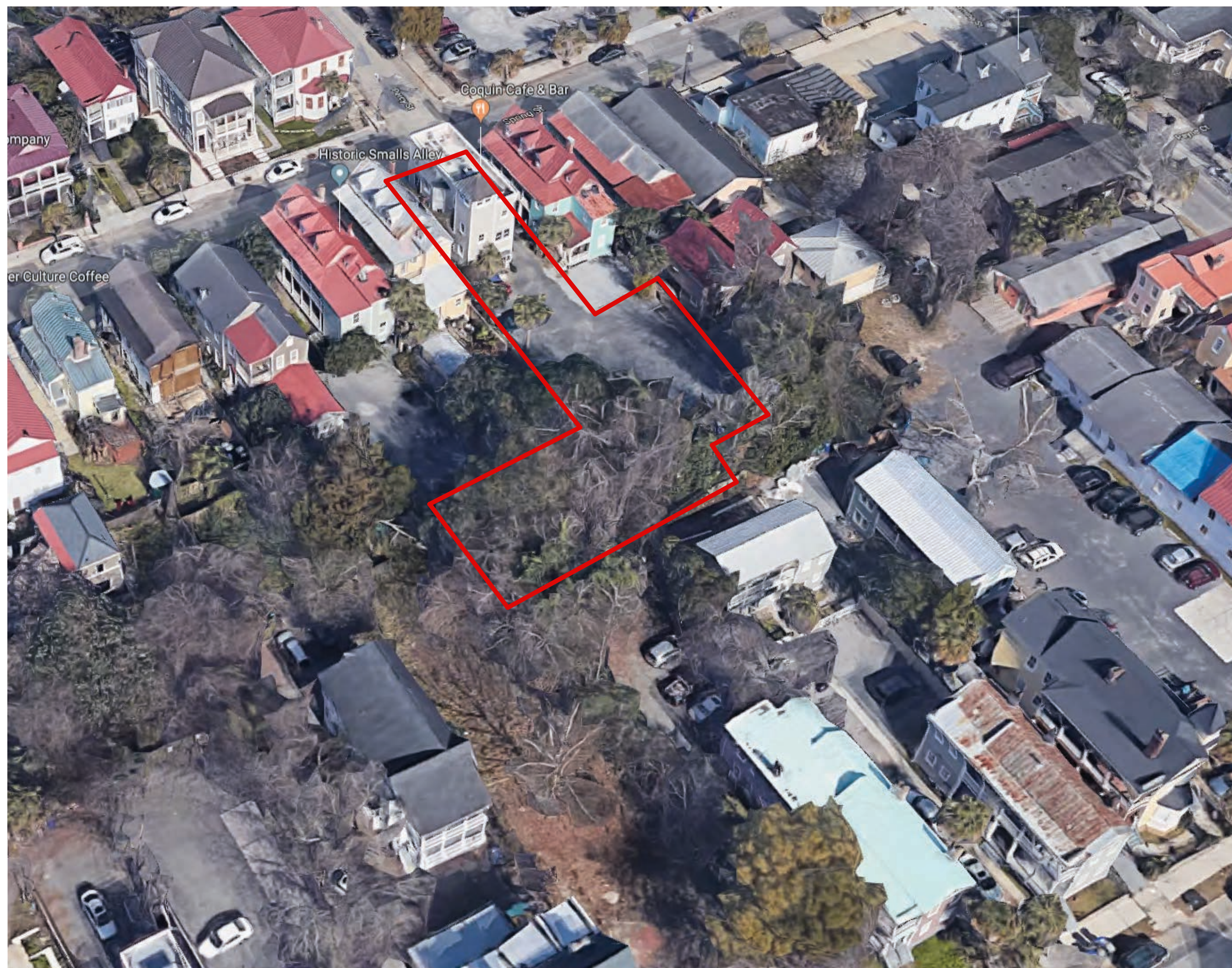
AERIAL VIEW: looking north
