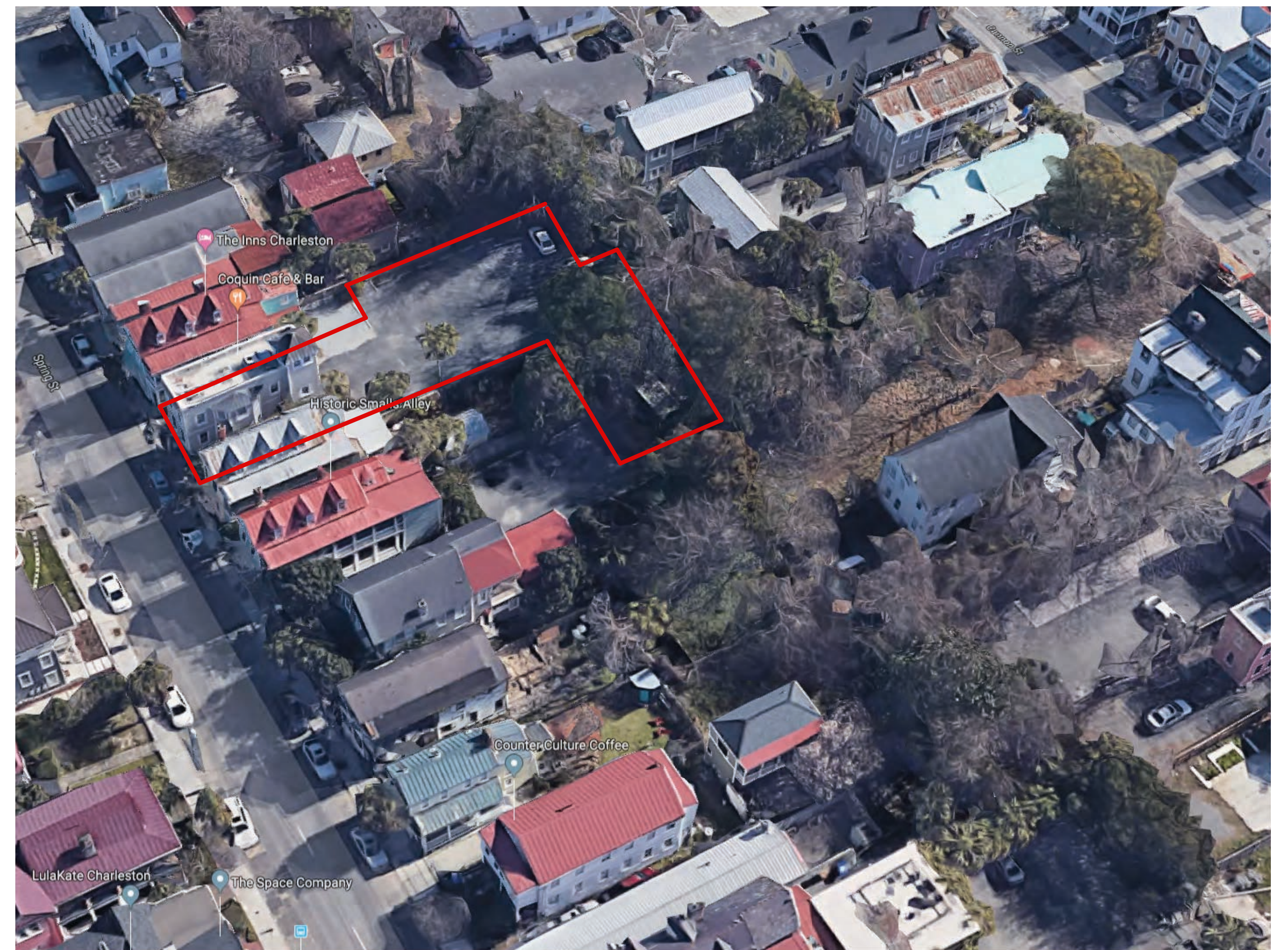
AERIAL VIEW: looking east
