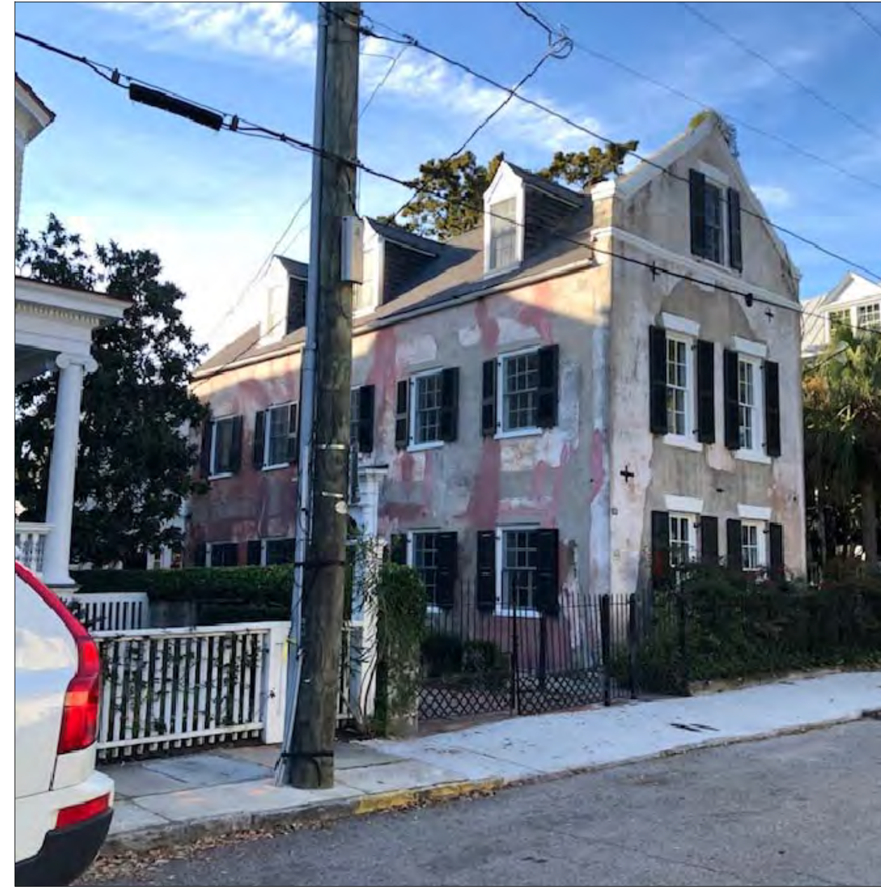
2. view of house looking northwest from Legare Street
