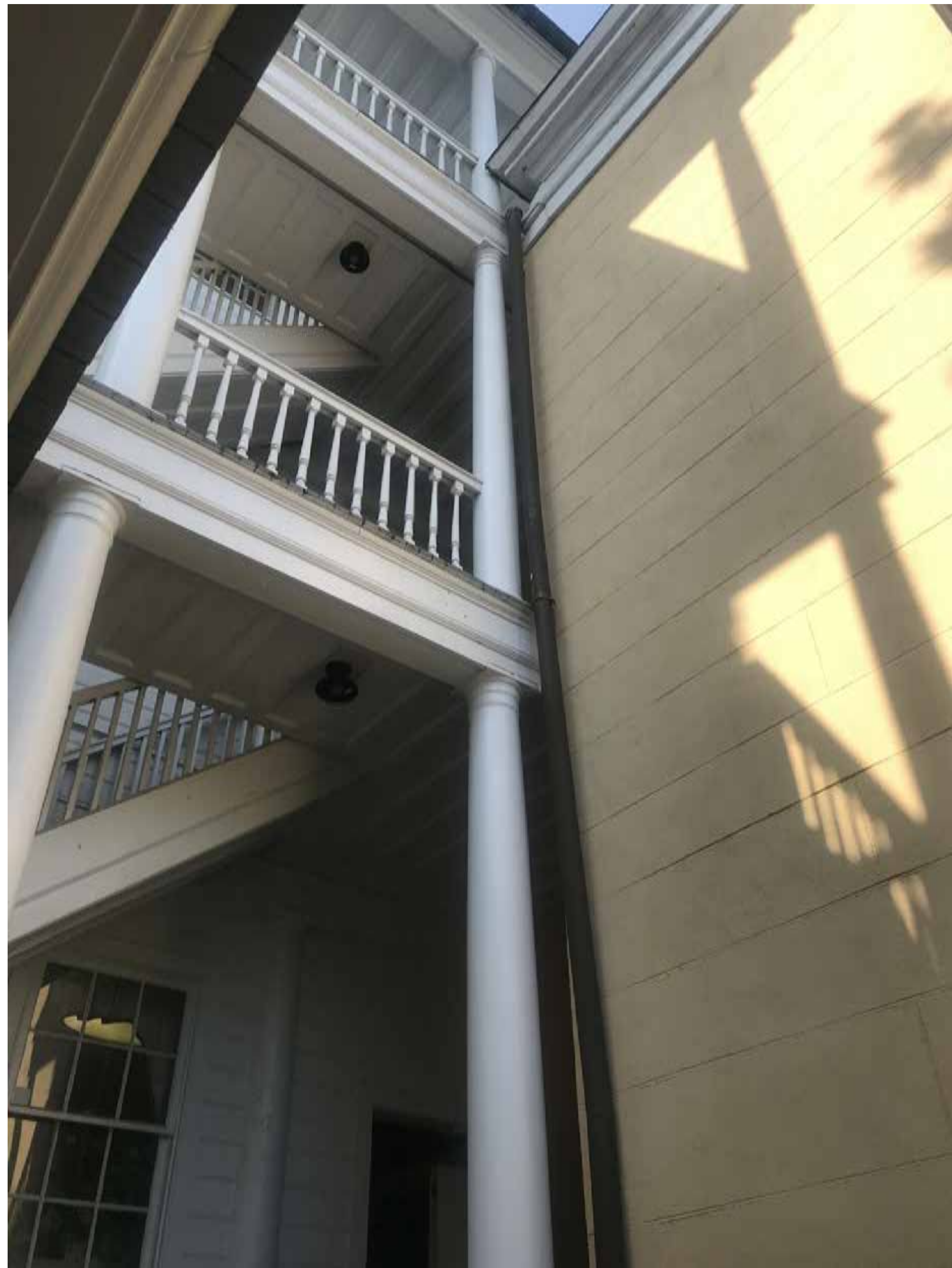
PHOTO 10: EXISTING VIEW OF PORCH AT REAR FROM CARRIAGE HOUSE
