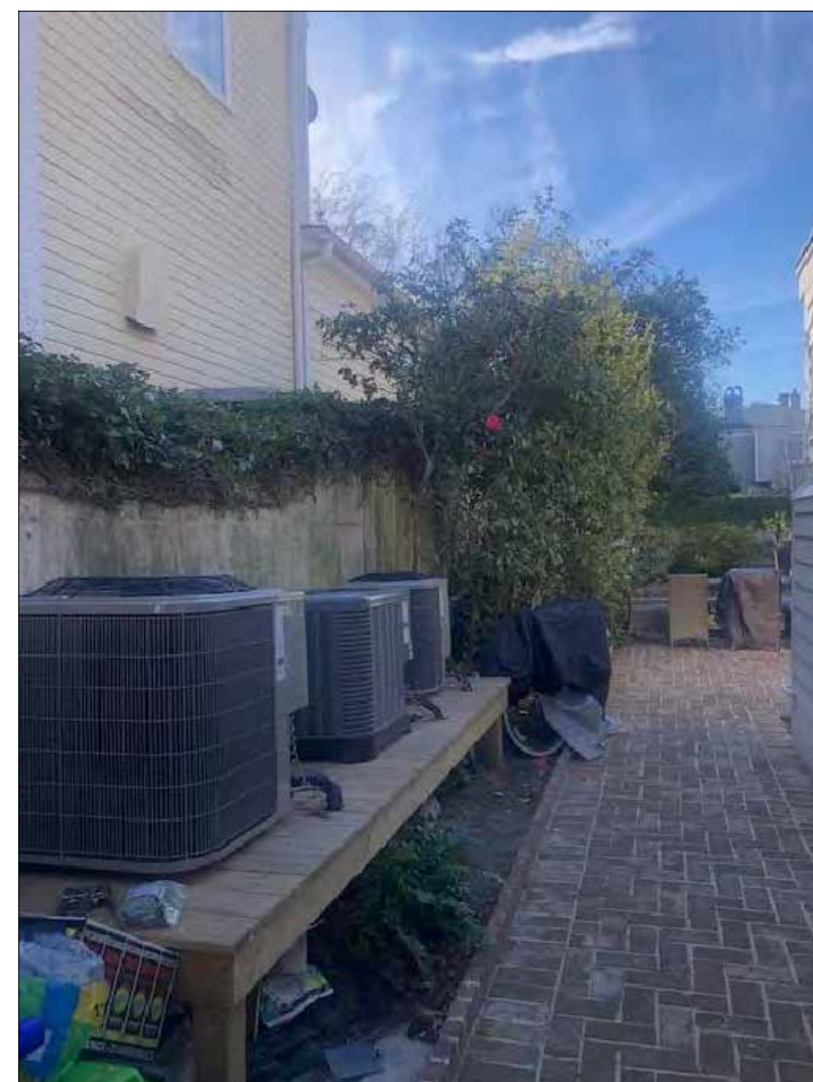
4. photo showing additional change in wall height
