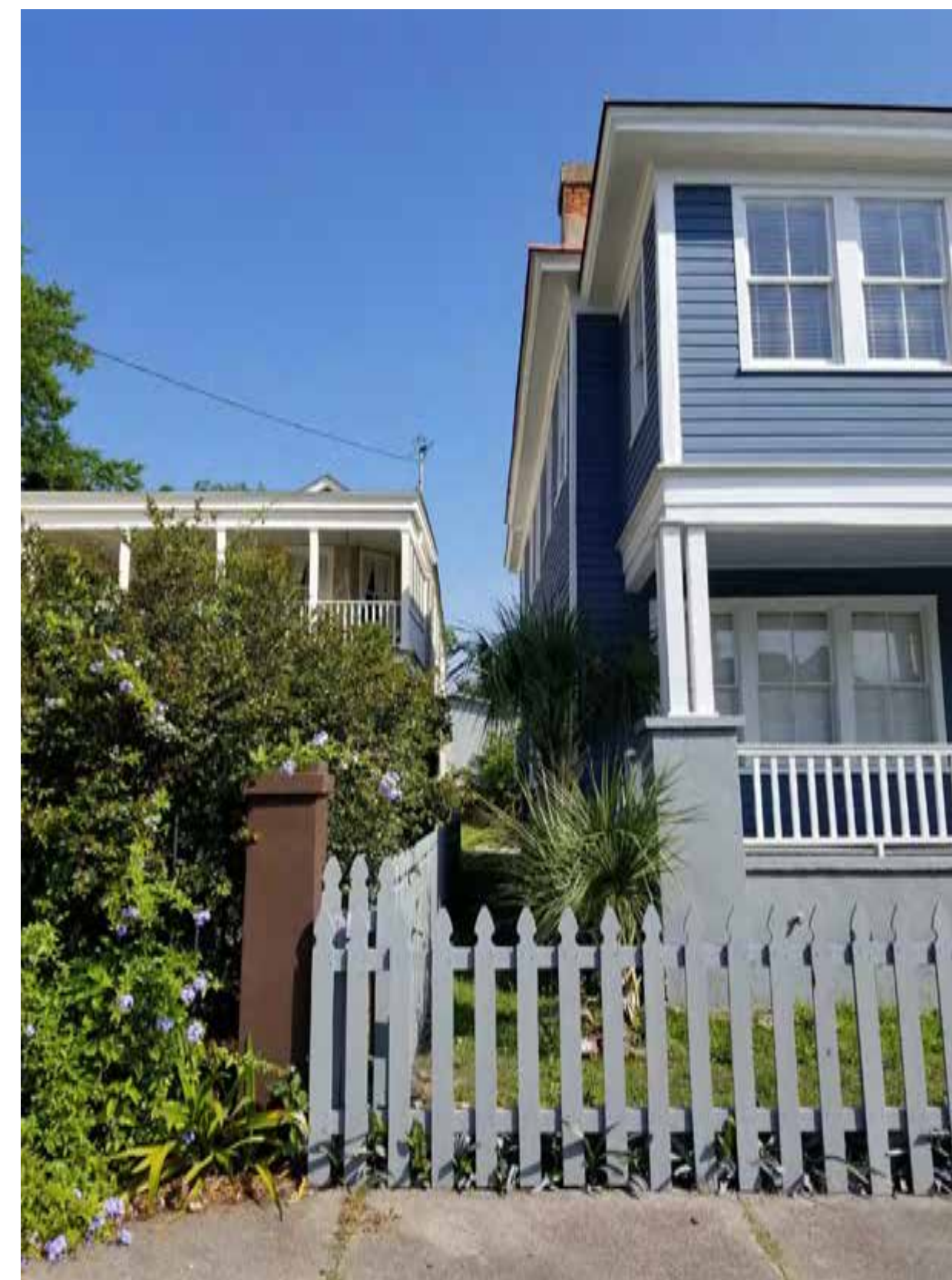
VIEW OF SOUTH WEST CORNER ELEVATION
