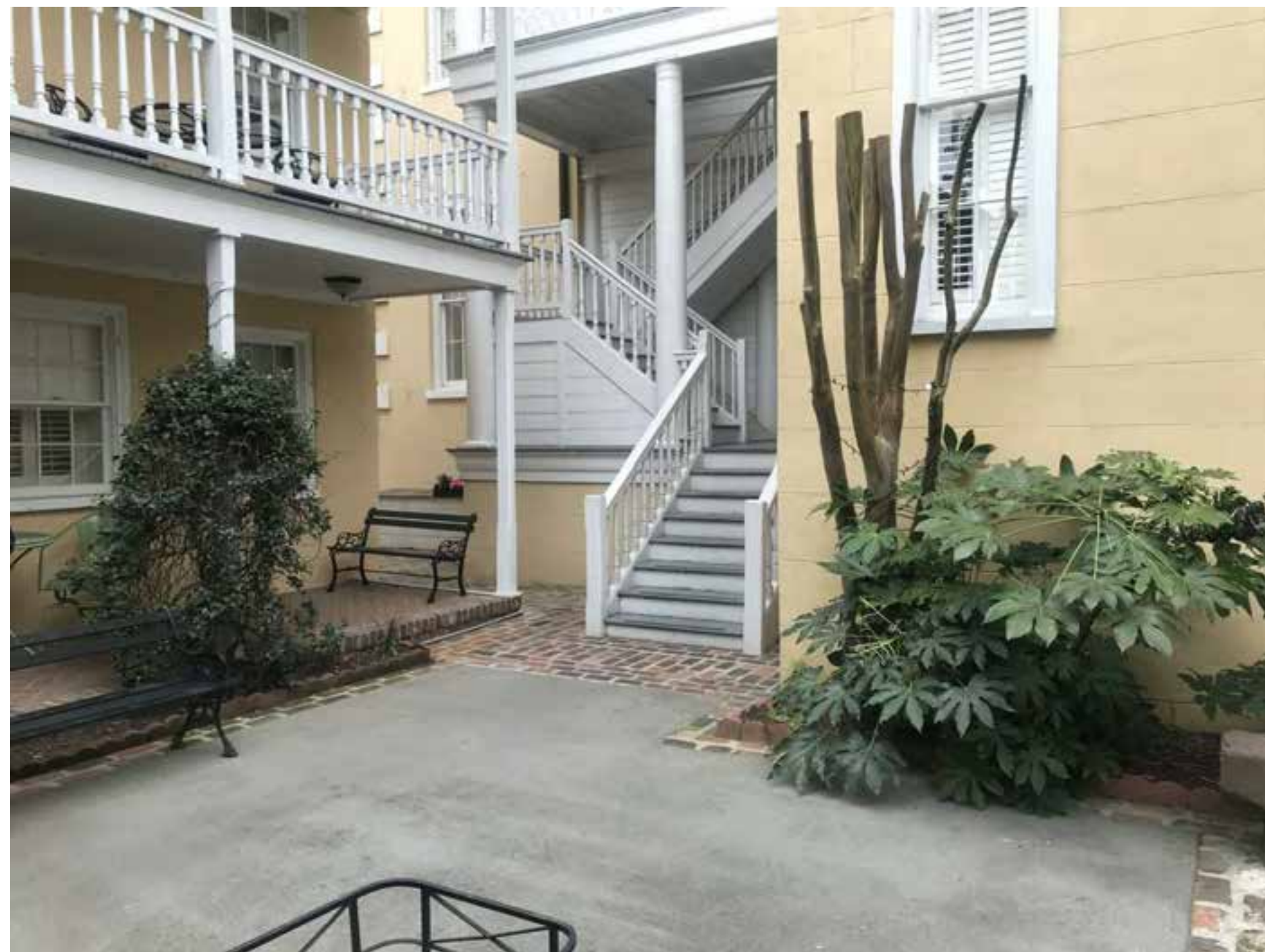
PHOTO 7: EXISTING VIEW OF PORCH/STAIRS FROM REAR PATIO
