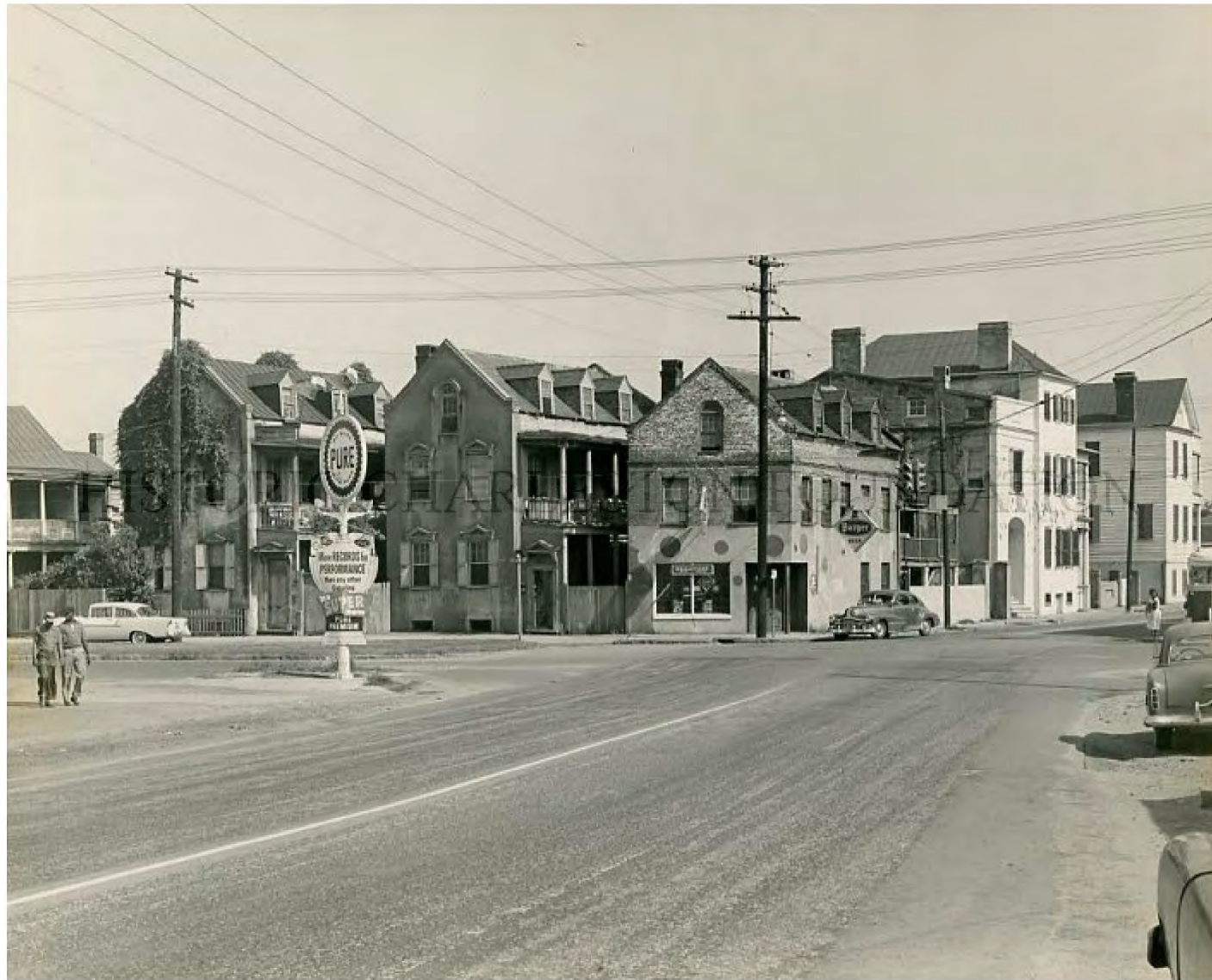
1963 HISTORIC PHOTO OF 41 CALHOUN STREET FROM EAST BAY STREET- DEMOLISHED 1964
