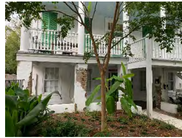
60 Spring Street - Masonry Piers at Ground Level
