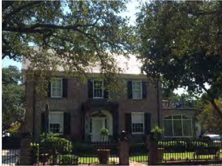
View of streetscape looking South. North elevation of 105 South Battery, rear chimney not visible.
