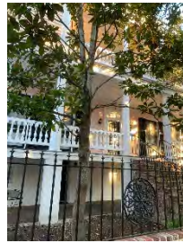
18 Montague Street - Masonry Piers at Ground Level
