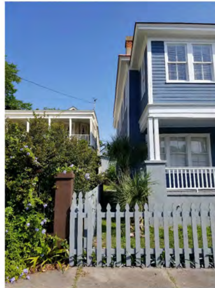
VIEW OF SOUTH WEST CORNER ELEVATION
