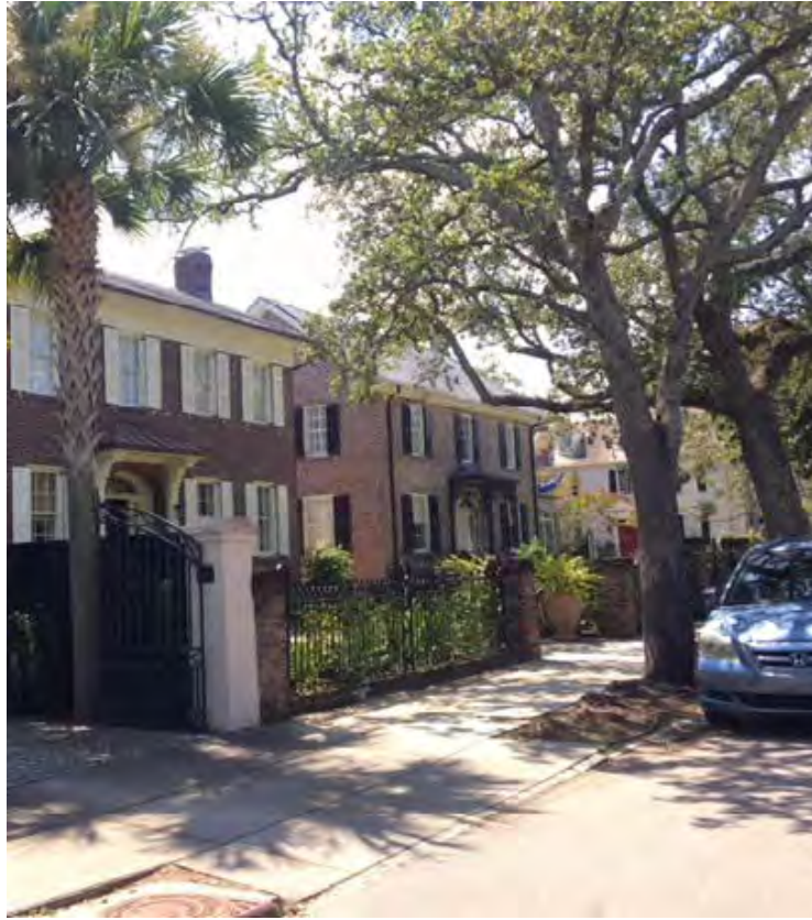
Northeast elevation of 105 South Battery. Rear chimney is not visible.
