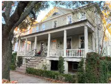
28 Montague Street - Masonry Piers at Ground Level
