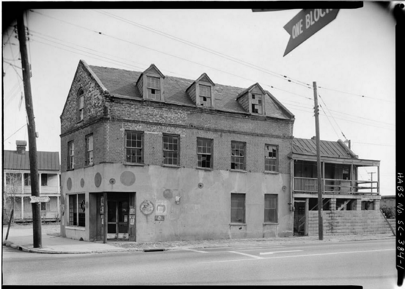
1963 HISTORIC PHOTO OF 41 CALHOUN STREET FROM EAST BAY STREET- DEMOLISHED 1964
