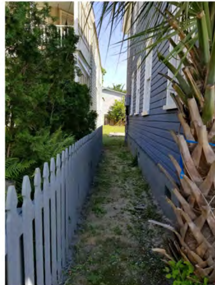
VIEW OF WEST SIDE ELEVATION FROM JUDITH STREET
