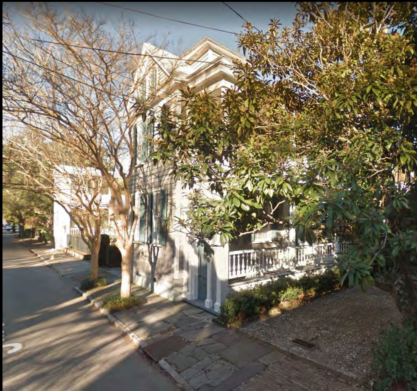
EXISTING SITE PHOTOS
