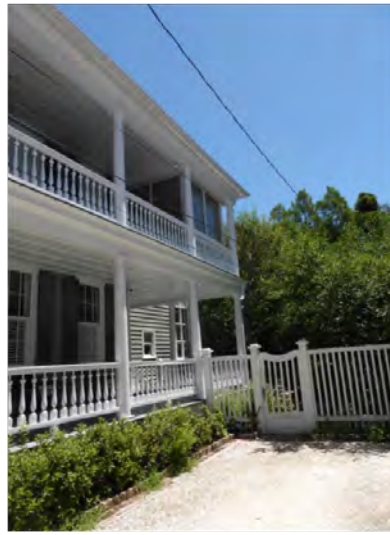
4 VIEW OF ADDITION FROM DRIVEWAY P-1 NO SCALE
