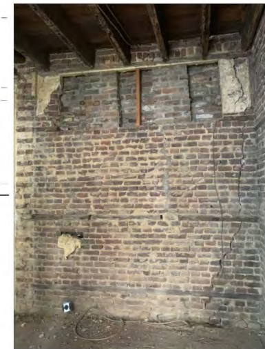
INTERIOR EVIDENCE OF ORIGINAL TRANSOM WINDOWS
