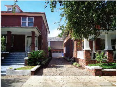
EXISTING SITE PHOTOS
