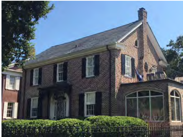
View of streetscape looking Southeast. Northwest view of 105 South Battery, rear chimney not visible.
