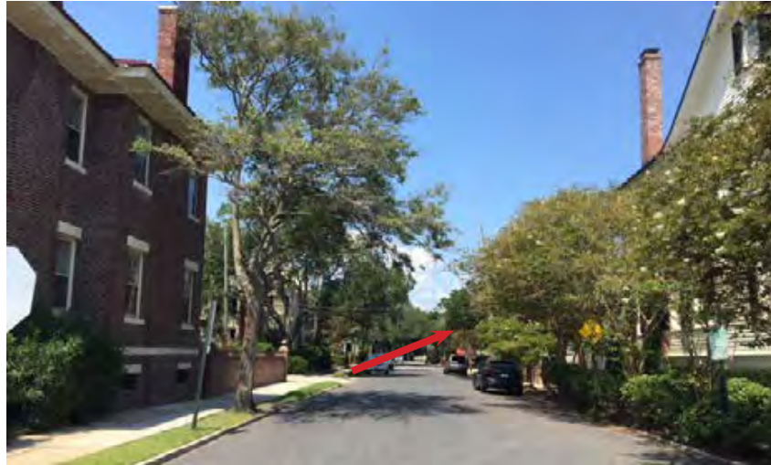
North view of Council Street streetscape. Location of 105 South Battery is shown by arrow.
