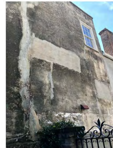
EXTERIOR EVIDENCE OF ORIGINAL TRANSOM WINDOWS
