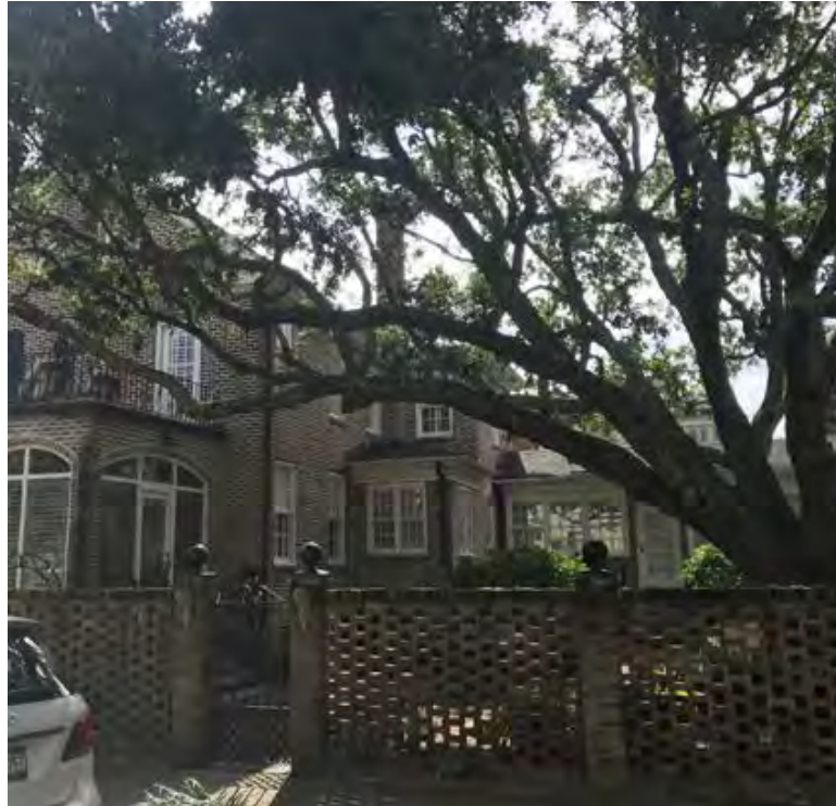
View of rear chimney from Council Street looking East. Same aspect of previous photo but approximately 20' further to the South.
