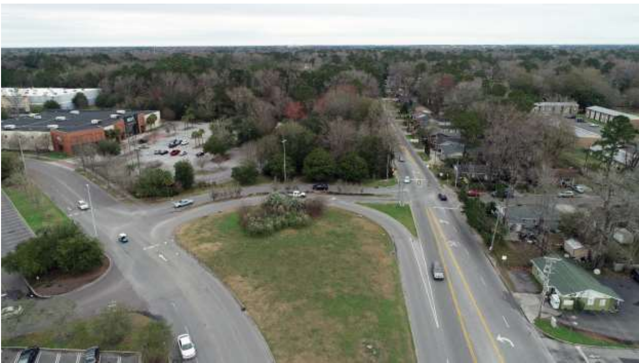
Figure I-4: Existing north entrance at Orleans Road.
