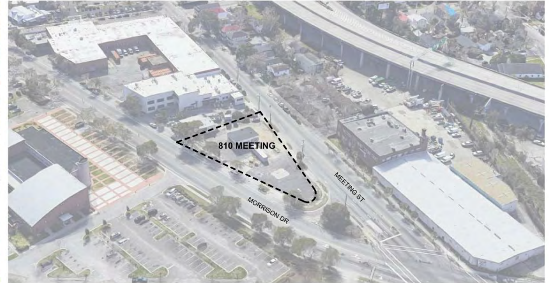
BIRD'S EYE PHOTO 2 - LOOKING SOUTH
