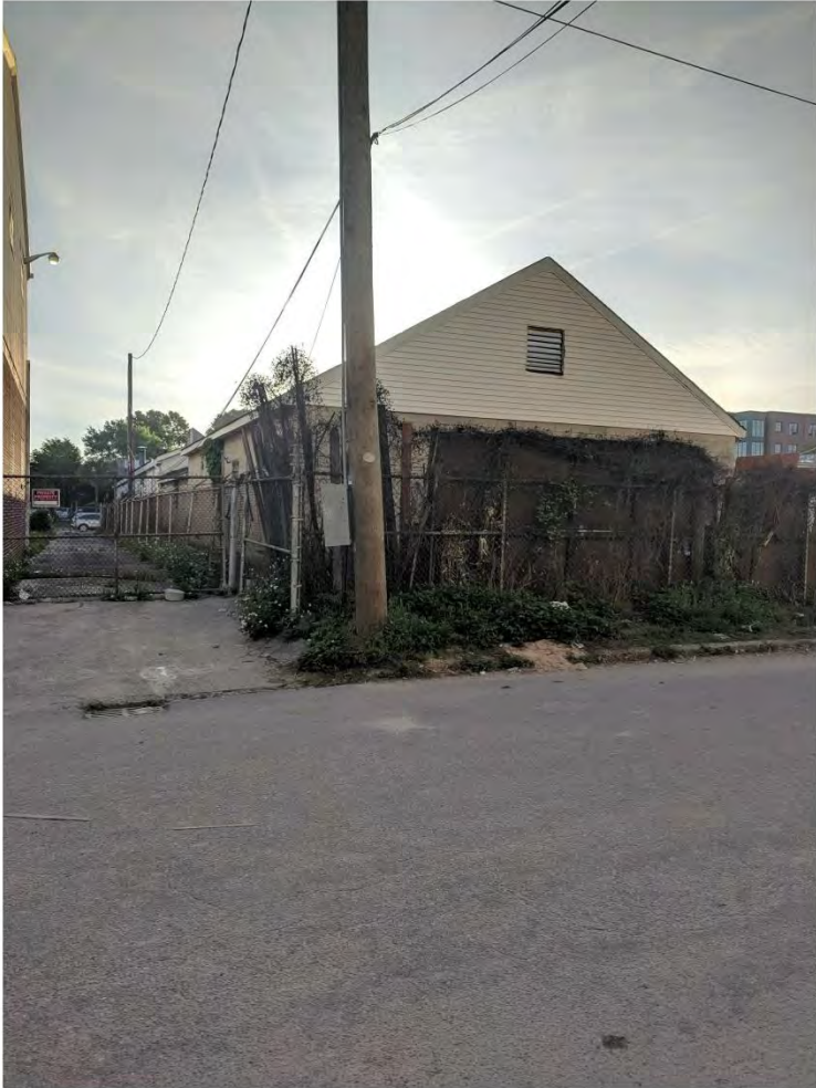
VIEW SOUTH ON WALNUT STREET
