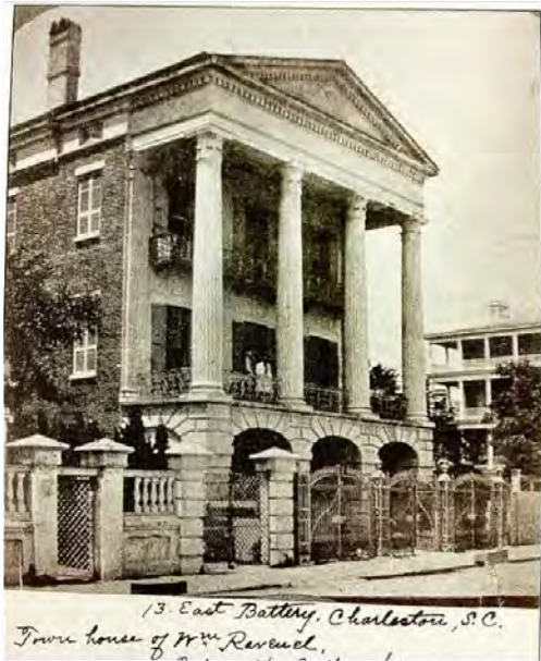
2 HISTORIC PHOTO—BEFORE EARTHQUAKE NO SCALE
