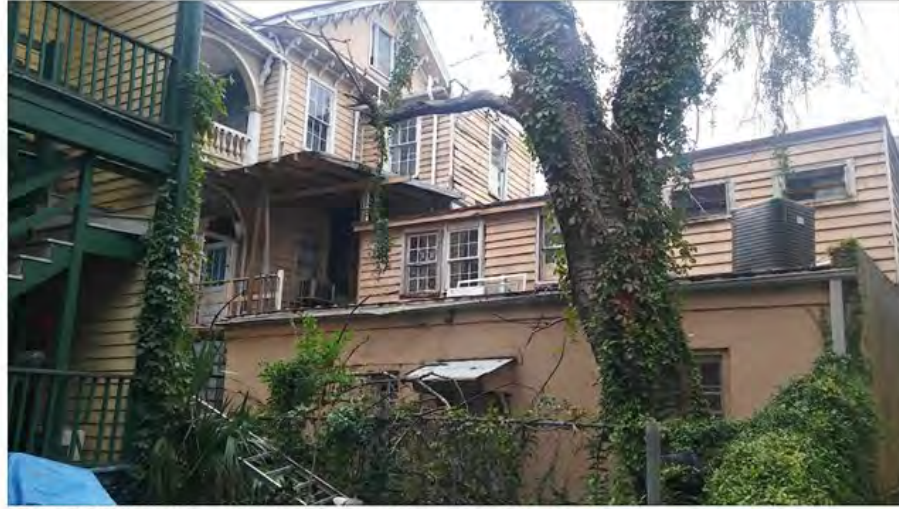
EAST END OF MAIN HOUSE: SERIAL ADDITIONS @ KITCHEN HOUSE (SOUTH ELEVATION)
