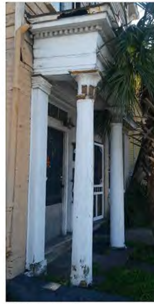
MAIN ENTRY PORTICO
