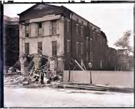
1 HISTORIC PHOTO—AFTER EARTHQUAKE NO SCALE
