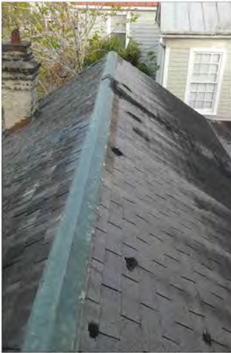
KITCHEN HOUSE ROOF (SLATE @ NORTH ONLY)
