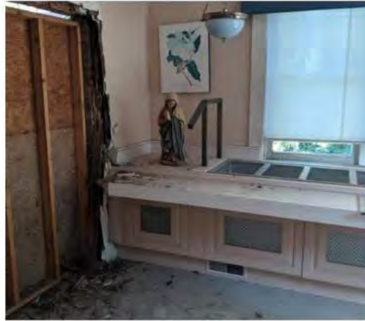
TEMPORARY WALL AT REAR ADDITION - BUFFET AREA
