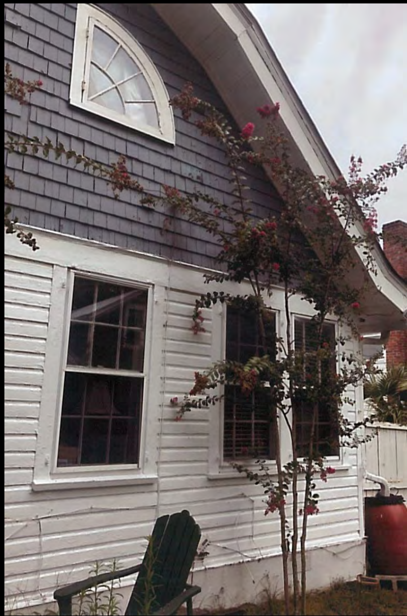
Area to be demolished
