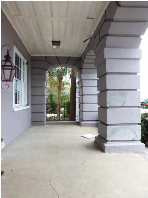
1 EAST BATTERY—PORCH FROM SOUTH A-3 NO SCALE
