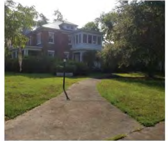
VIEW OF SITE FROM CORNER
