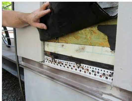
LACK OF DRAINAGE MAT & WEEP SCREED
