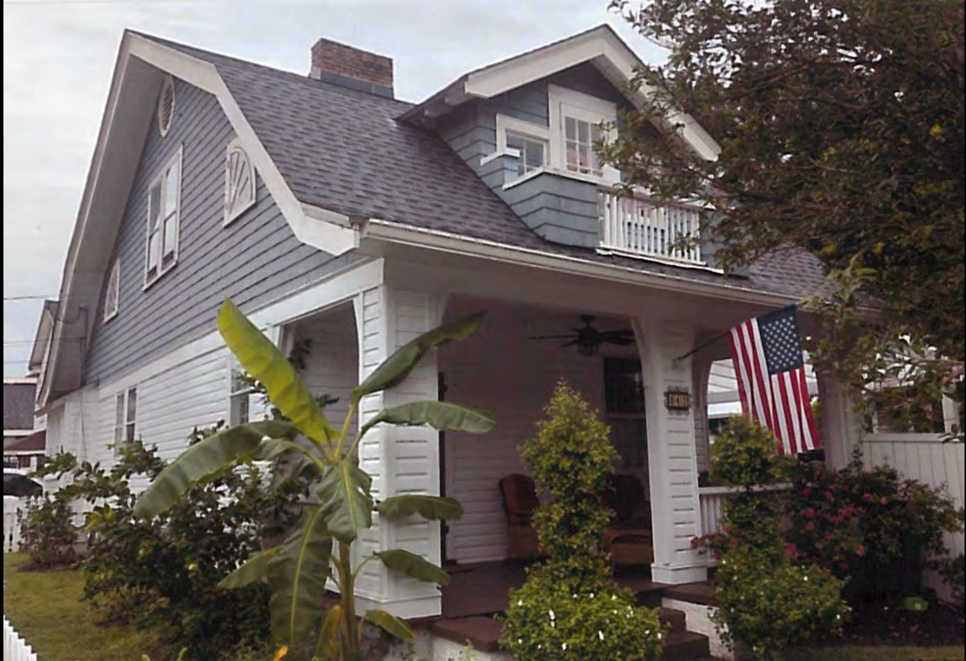
North and West Elevations
