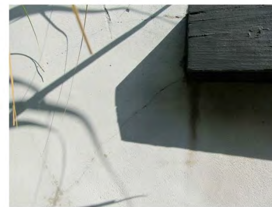
DEFFICIENT CONTROL JOINT PLACEMENT
