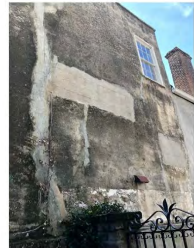
EXTERIOR EVIDENCE OF ORIGINAL TRANSOM WINDOWS
