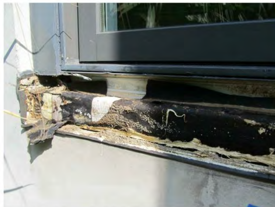
IMPROPER SILL CONFIGURATION
