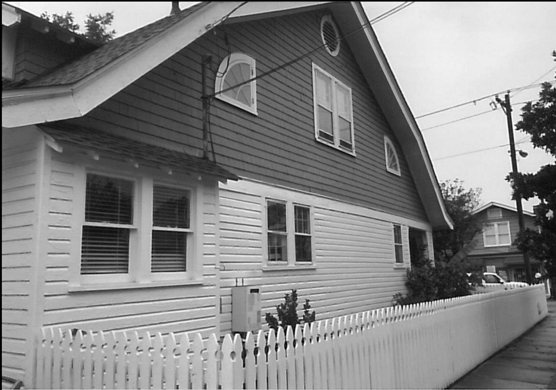
North Elevation – along Maple Street
