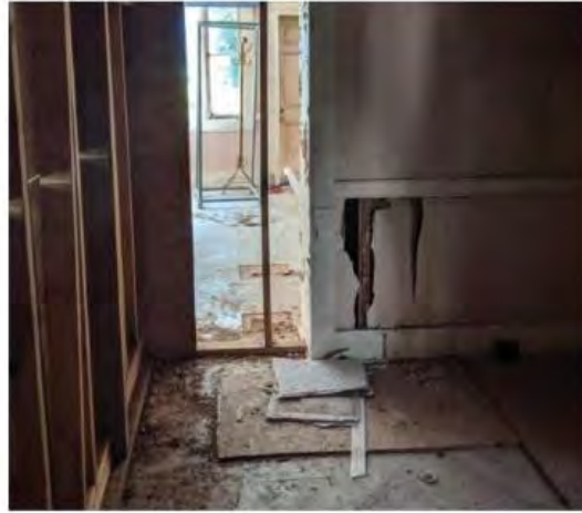
TEMPORARY WALL AT REAR ADDITION
