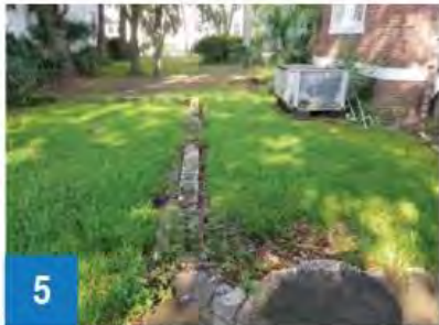
5 REMAINS OF PREVIOUSLY DEMOLISHED ACCESSORY BUILDING
