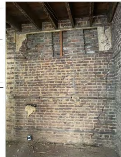
INTERIOR EVIDENCE OF ORIGINAL TRANSOM WINDOWS
