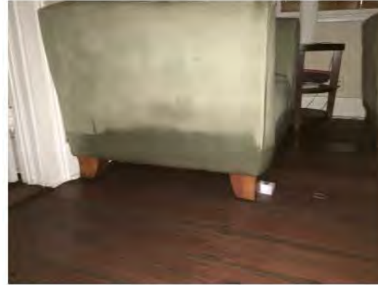
INTERIOR SHOWING WATER LEVEL
