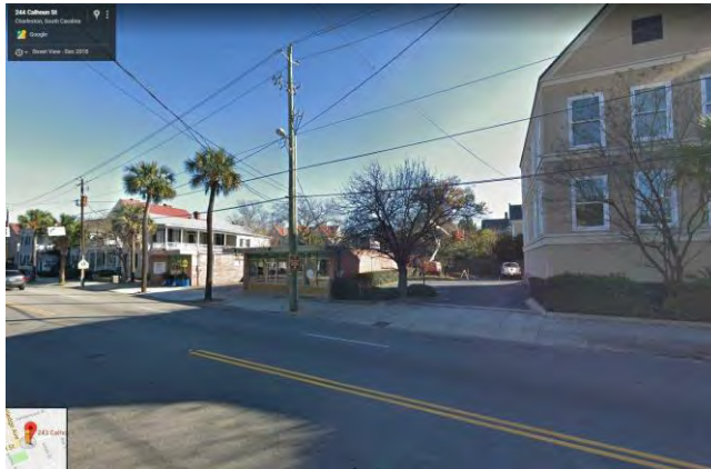
EXISTING WEST FACADE
