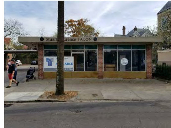
EXISTING NORTH FACADE
