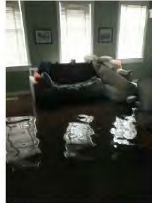
INTERIOR SHOWING FLOODING
