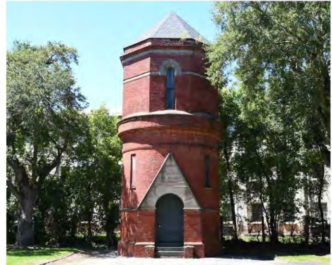
Water tower + artesian well, 1887
