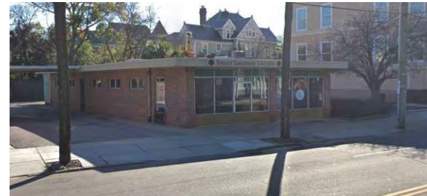
EXISTING EAST FACADE
