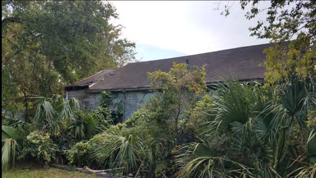
Left side of the house
