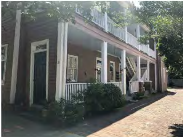
SOUTHWEST CORNER SHOWING PIAZZA SCREEN
