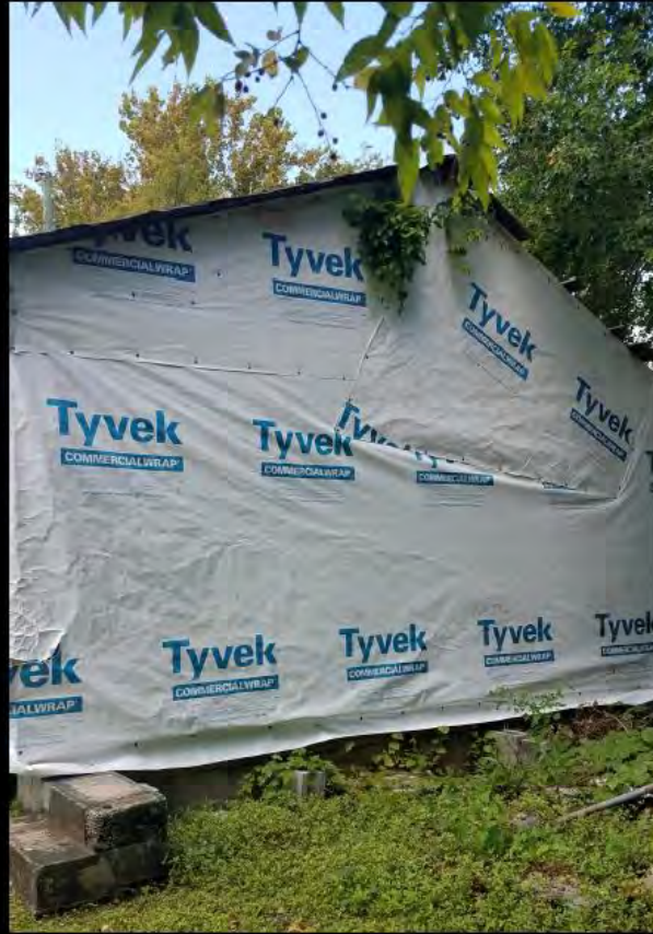
Rear of the house
