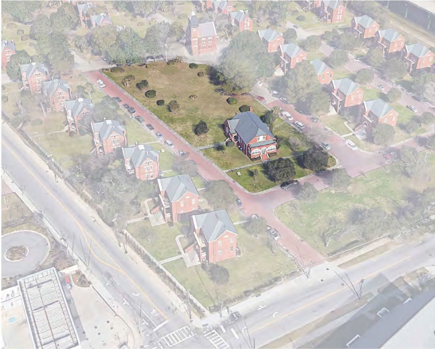
CURRENT SITE AERIAL LOOKING NORTH EAST
