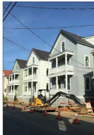
ADJACENT STRUCTURES @ AMHERST ST
