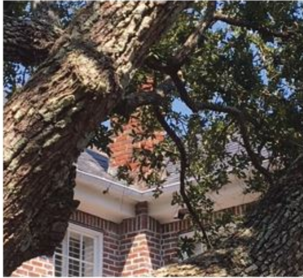
Detailed view of chimney situated at roof valley. Streetscape view of chimney is obstructed by tree.
