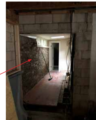
Interior of existing masonry wall
