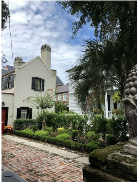
View from East Bay Street looking north-east towards (south) side facade.
