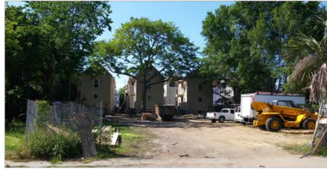
EXISTING SITE (AMHERST STREET 'SISTER HOUSES' UNDER CONSTRUCTION IN BACKGROUND)
