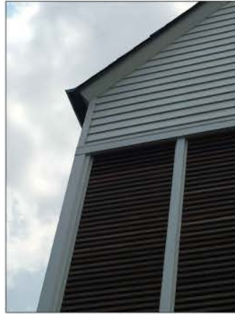
LOUVERED SCREEN ELEMENT (but painted)
