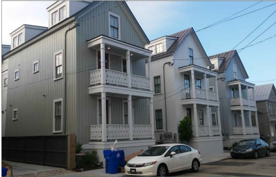
ADJACENT STRUCTURES @ AMHERST ST
