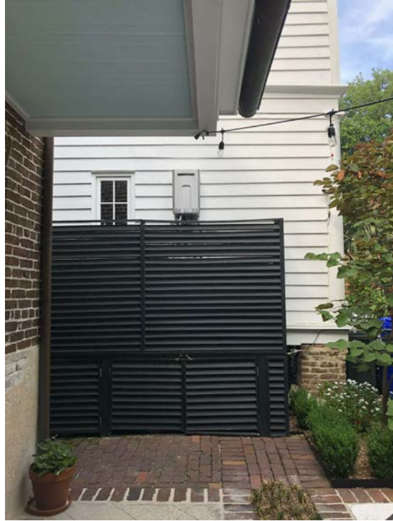
View from courtyard looking east towards rear (west) facade.
