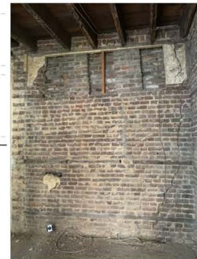
INTERIOR EVIDENCE OF ORIGINAL TRANSOM WINDOWS
