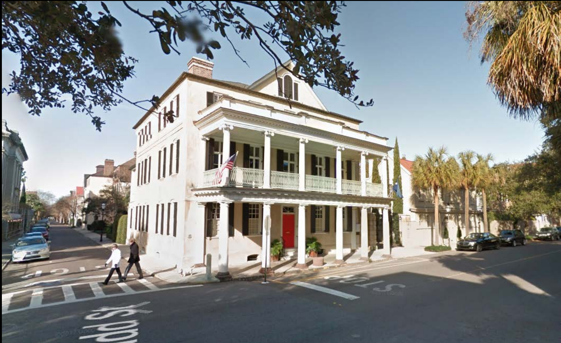
EXISTING SITE PHOTOS
