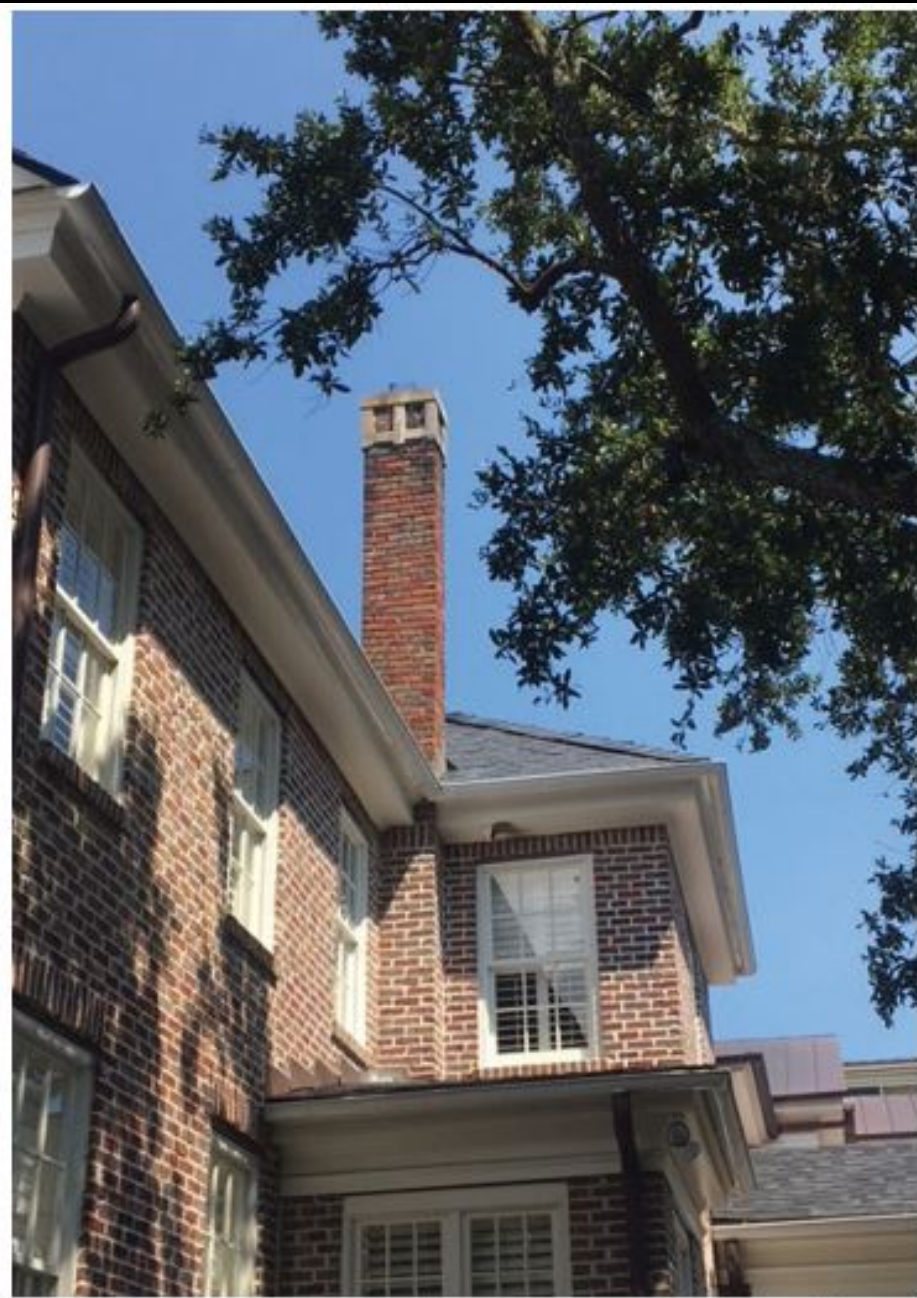
View of chimney at roof valley located at the intersection of the South and West elevations. Photo taken standing at backyard fence.
