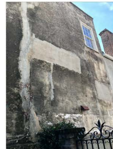
EXTERIOR EVIDENCE OF ORIGINAL TRANSOM WINDOWS
