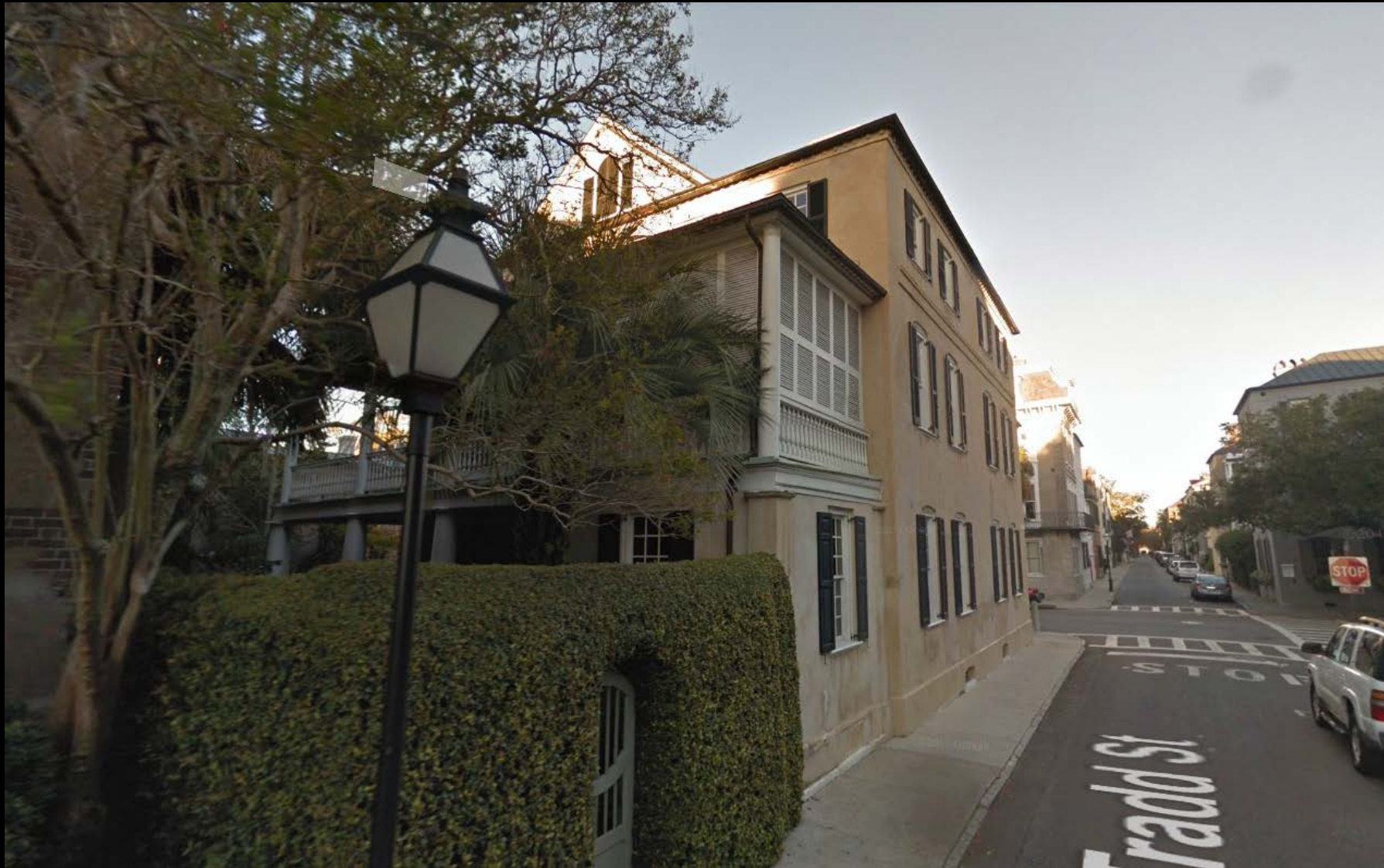
EXISTING SITE PHOTOS
