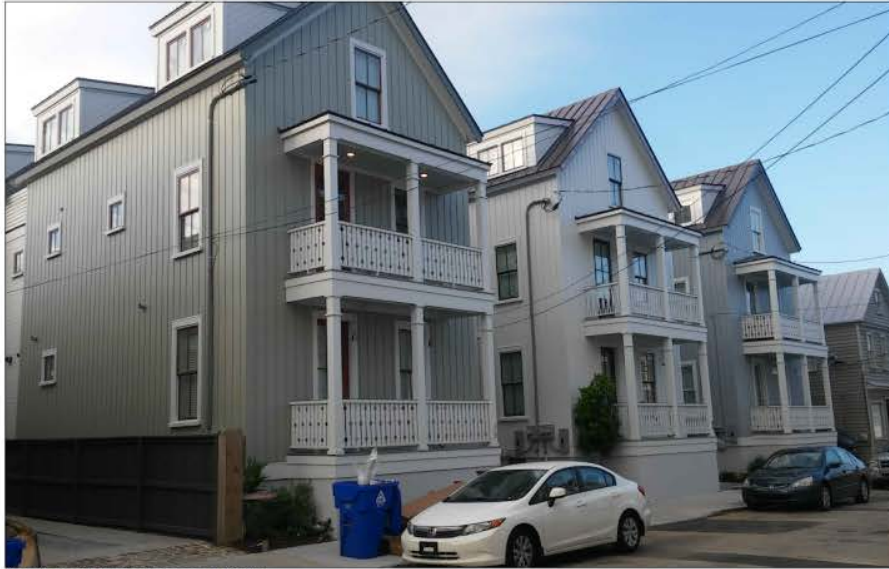
ADJACENT STRUCTURES @ AMHERST ST
