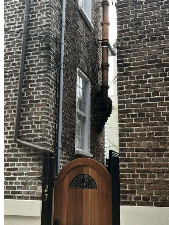
View from Hasell Street looking south towards NE corner of primary building and area of kitchen addition.
