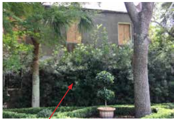
Existing windows behind shrubs
