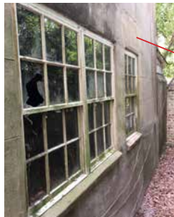
Existing windows to be replaced
