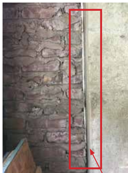
Existing gap between old and new
