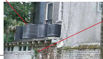
Removal of HVAC placement
