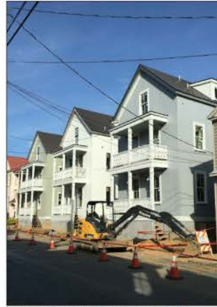
ADJACENT STRUCTURES @ AMHERST ST
