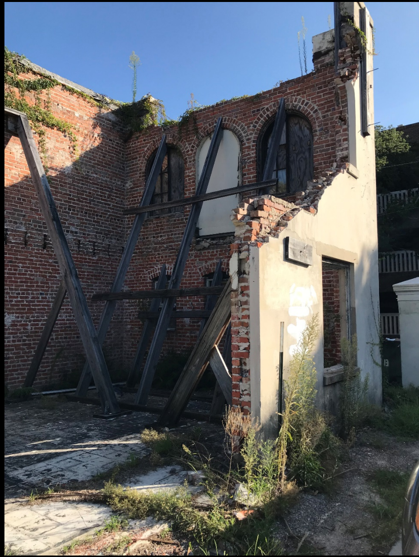
EXISTING SITE PHOTOS
