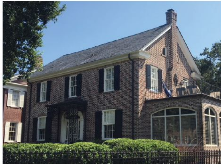
View of streetscape looking Southeast. Northwest view of 105 South Battery, rear chimney not visible.
