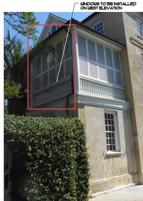
3 ENCLOSURE DETAIL A-2 NO SCALE
