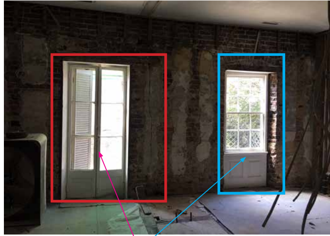
Replace existing window with existing central door
