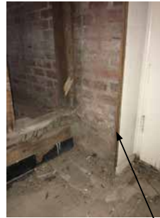
Original height of flooring
