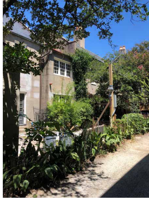
South Elevation looking North East
