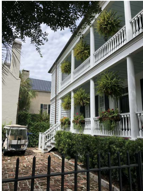
View from East Bay Street looking east towards (south) side facade.
