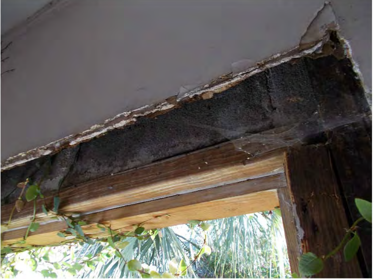
Figure 10: another example of a window surround
