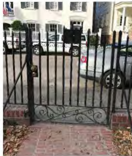
Existing wrought iron pedestrian gate
