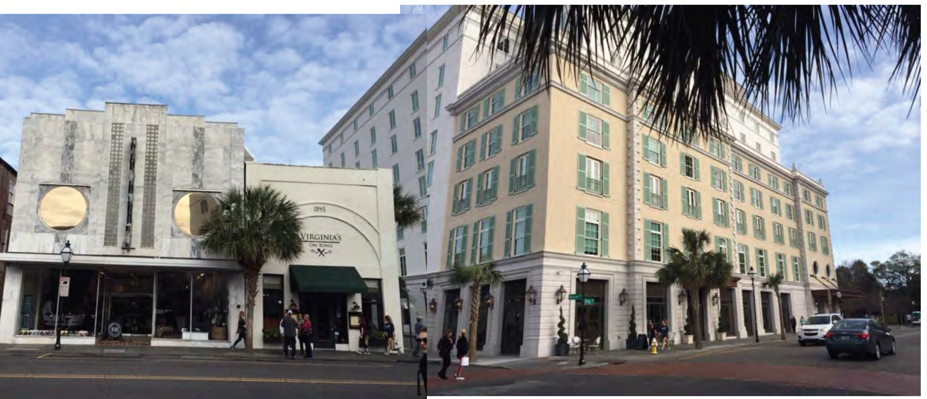
King Street East Elevation
