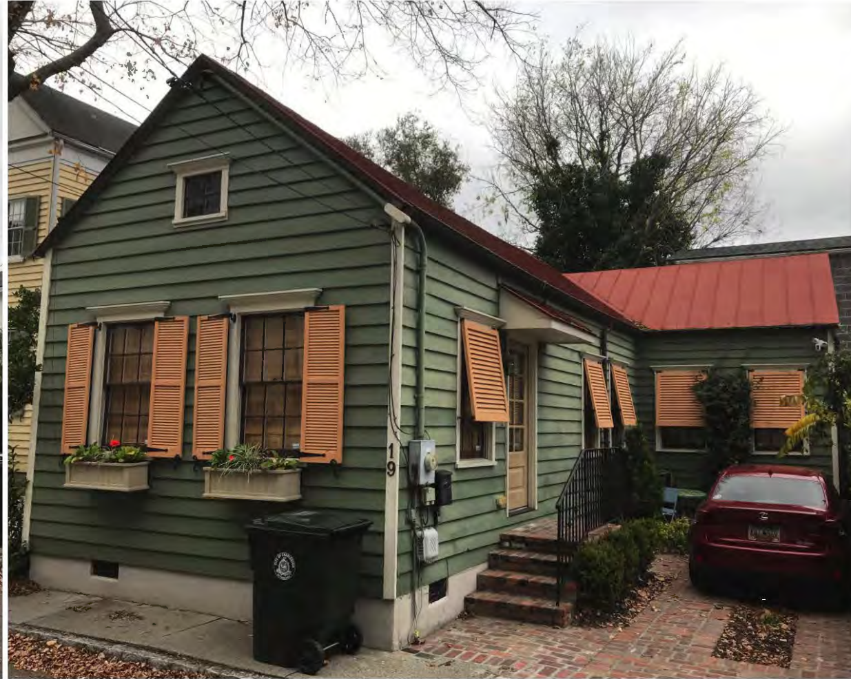
2 EXISTING NW CORNER
