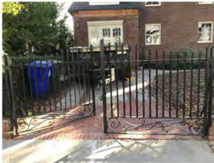
Existing wrought iron drive gate
