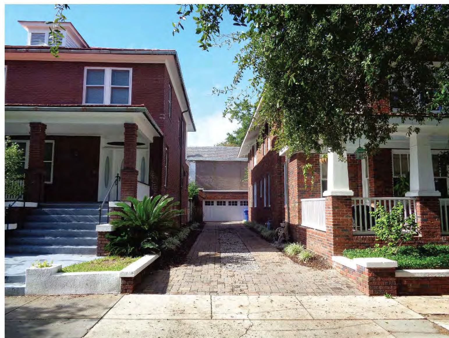
EXISTING SITE PHOTOS
