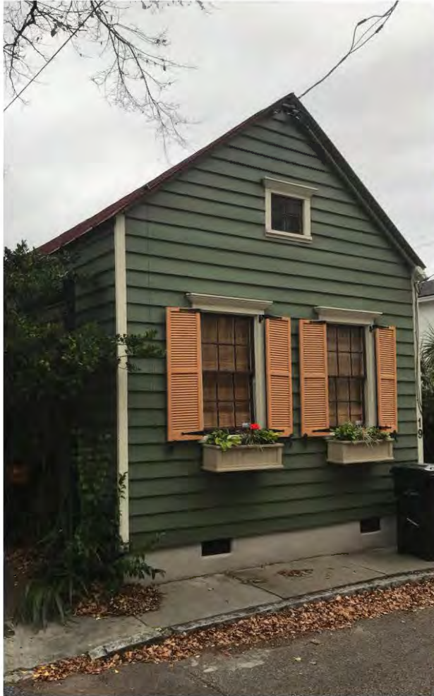
1 EXISTING NE CORNER
