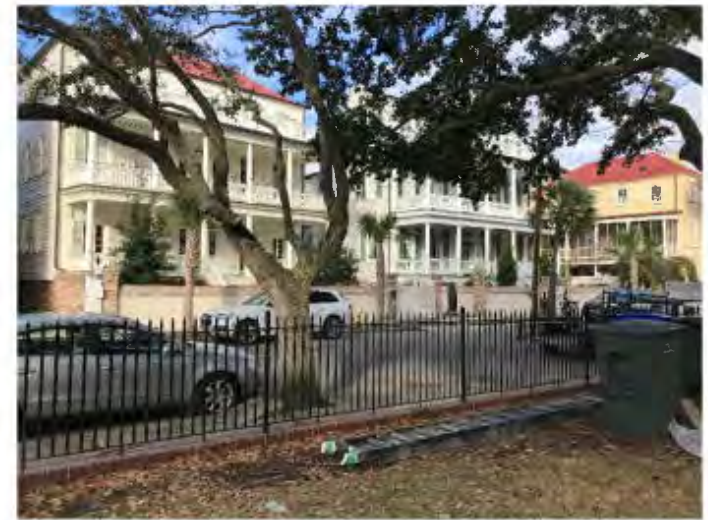
Existing coping wall and wrought iron pedestrian gate. Background: 44 and 46 SB
