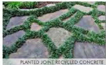
PLANTED JOINT RECYCLED CONCRETE
