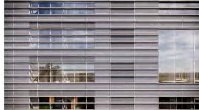
WEST ELEVATION WALL
