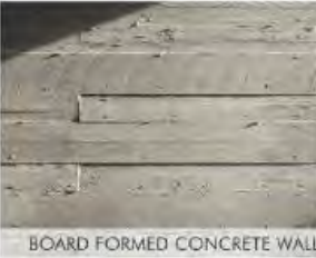
BOARD FORMED CONCRETE WALL
