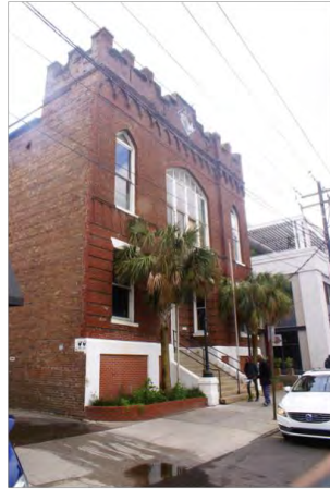
north east corner from calhoun street
