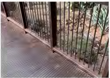
MONICOLS PERFORATED METAL, 1/16" ROUND ON 3/32" STAGGERED CENTERS WITH SOLID MARGINS ON ALL SIDES FOR BRIDGES AT RAIN GARDEN/ INFILTRATION AREAS AT R.O.W. IMAGE FOR REFERENCE ONLY. FINAL MATERIAL COLOR TO MATCH BUILDING ELEMENTS AND NOT CORTEN STEEL.
