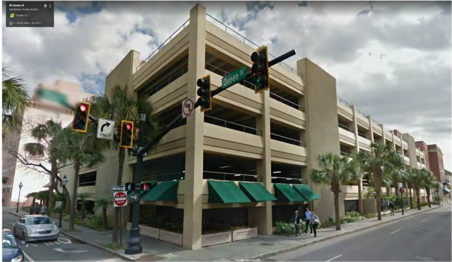
Parking Garage Across King Street
