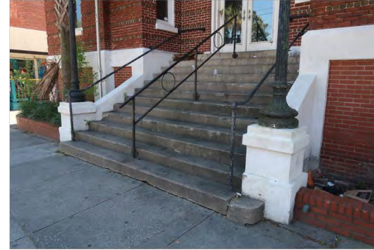
front steps from north west
