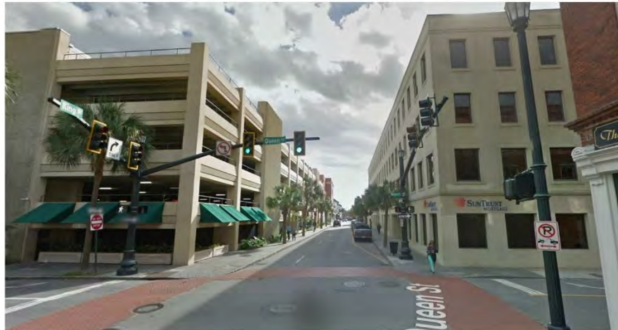
King Street - Looking South
