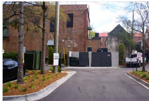
west elevation - adjacent property dumpster enclosure
