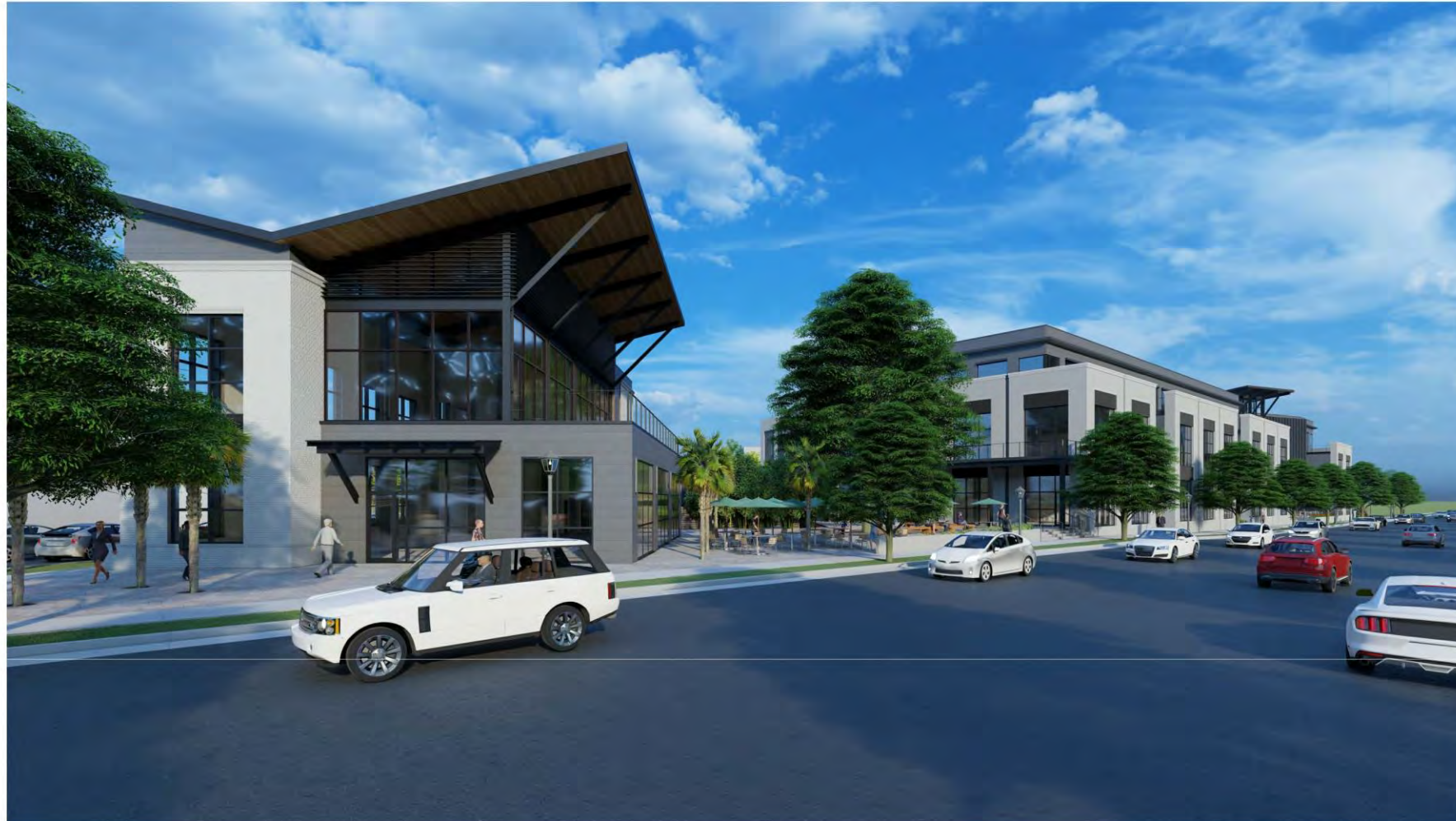
PERSPECTIVE FROM BRIGADE ST. AND MORRISON DR. LOOKING EAST TOWARDS MAIN ENTRANCE - CURRENT PROPOSAL
