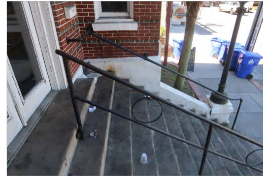
front steps from landing looking down to sidewalk
