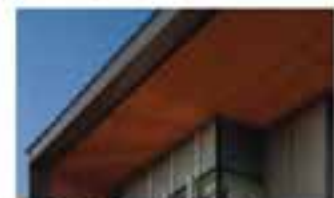
WOOD SOFFIT ACCENTS
