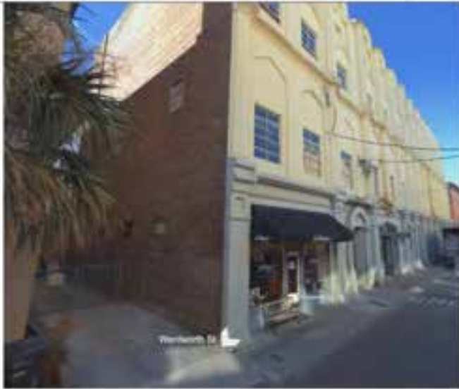
EAST FACADE AT WENTWORTH STREET
