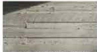
BOARD FORMED CONCRETE WALL
