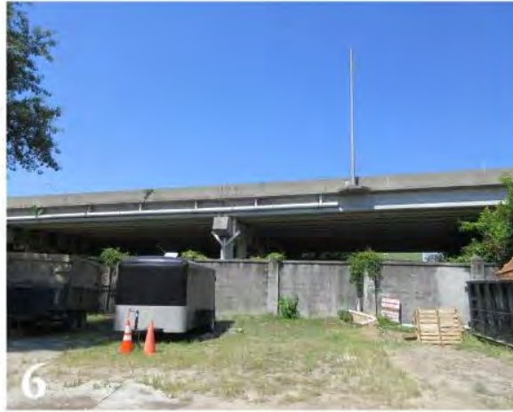
6 Elevated I-26 highway along the western boundary of the site.
