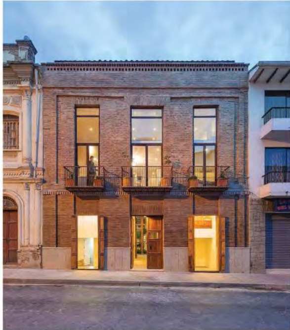
Large scale openings within a simple facade composition.
