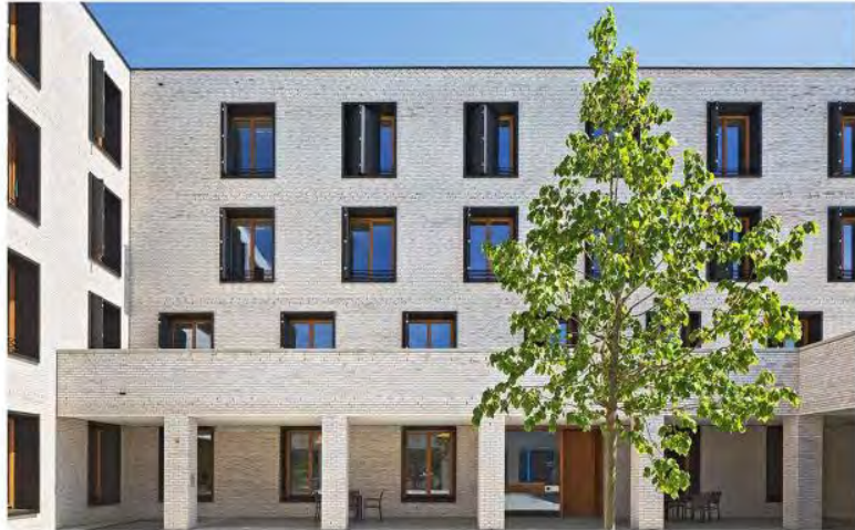
An orderly arrangement of deeply set openings creates a strong play of light and shadow.
