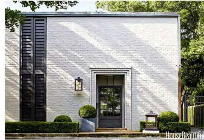
Articulated brick detailing around openings in an otherwise minimal facade.
