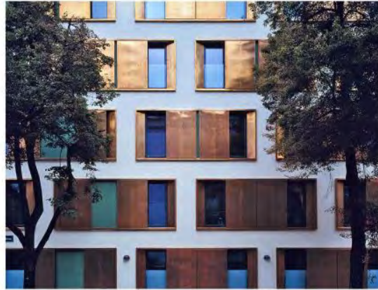
Playful arrangement of windows with copper surrounds.
