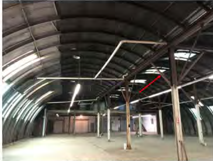
Picture 3 –Knee braces at columns
