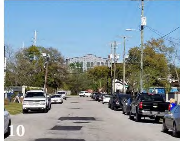
10 Terminated view at the opposite end of Williman Street at Foundry Point.
