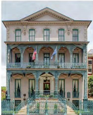
John Rutledge House, Charleston, SC
