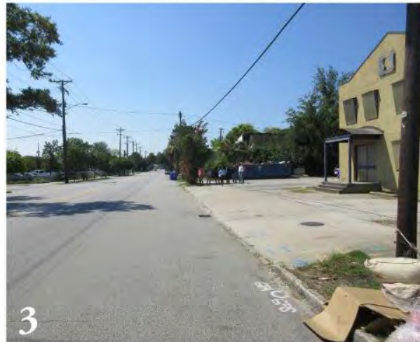
3 The Meeting Street frontage is a continuous curb-cut with no defined sidewalk.
