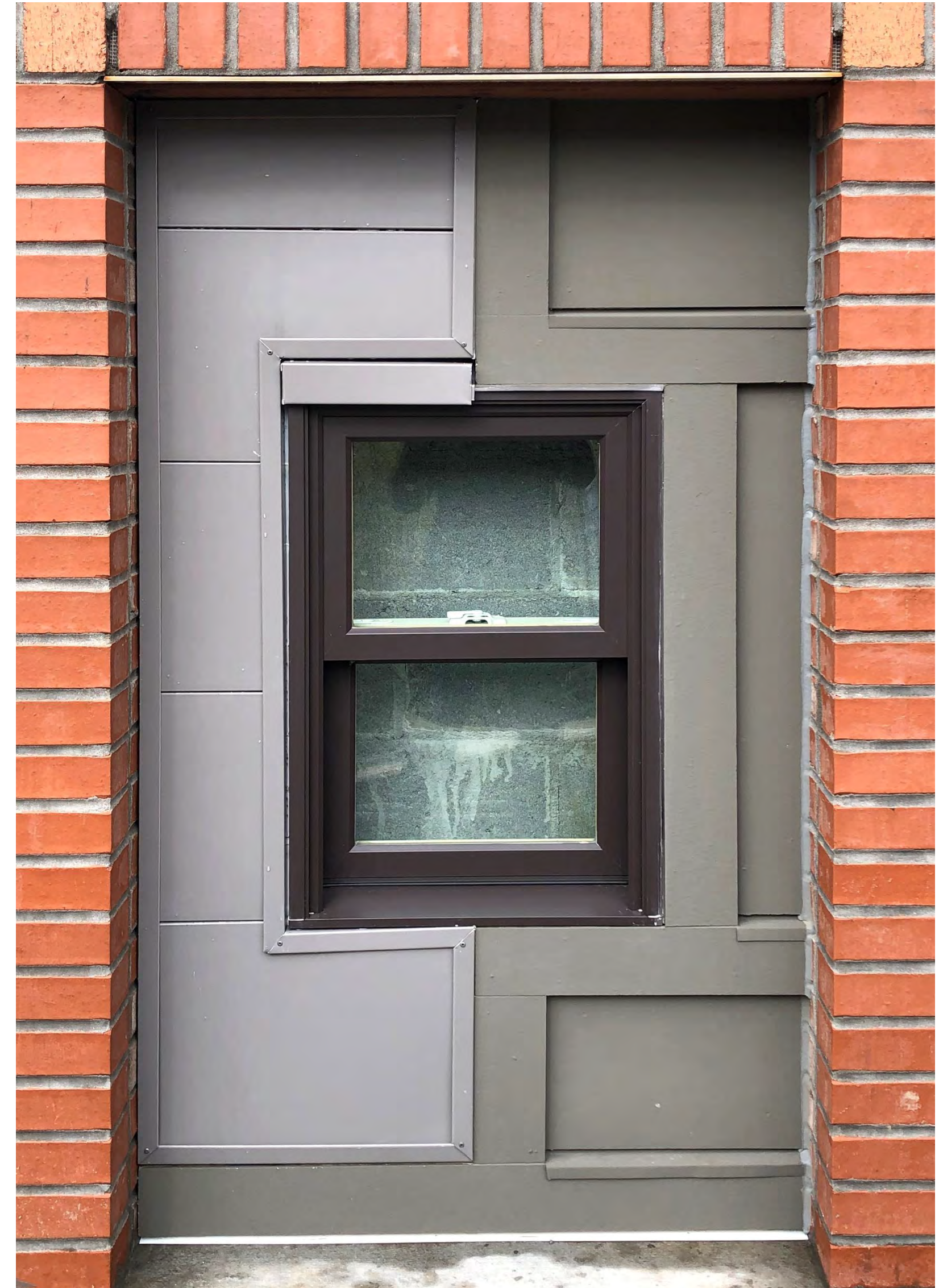
Material options for North Elevation window bays: Metal panel (left, requested by BAR) vs. Fiber cement panel (right, preferred by applicant)
