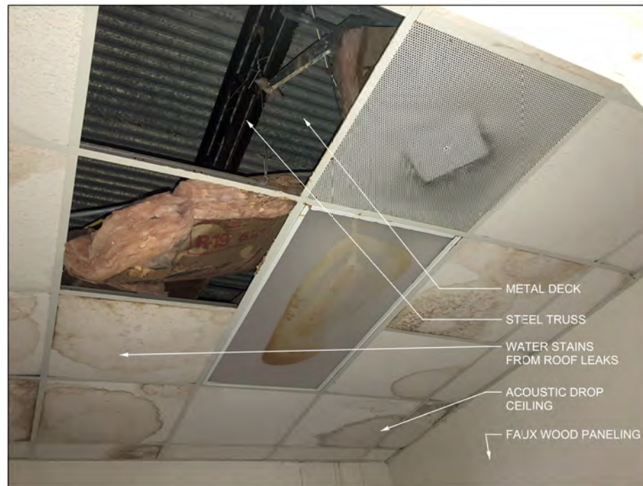
DROP CEILING WITH ROOF STRUCTURE BEYOND
