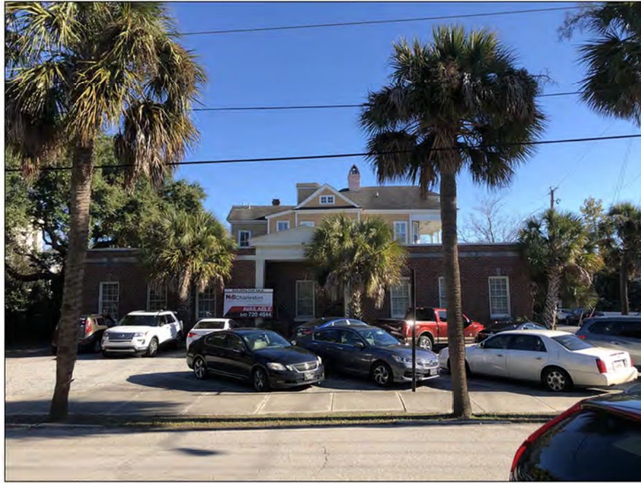
FRONT GADSDEN STREET FACADE
