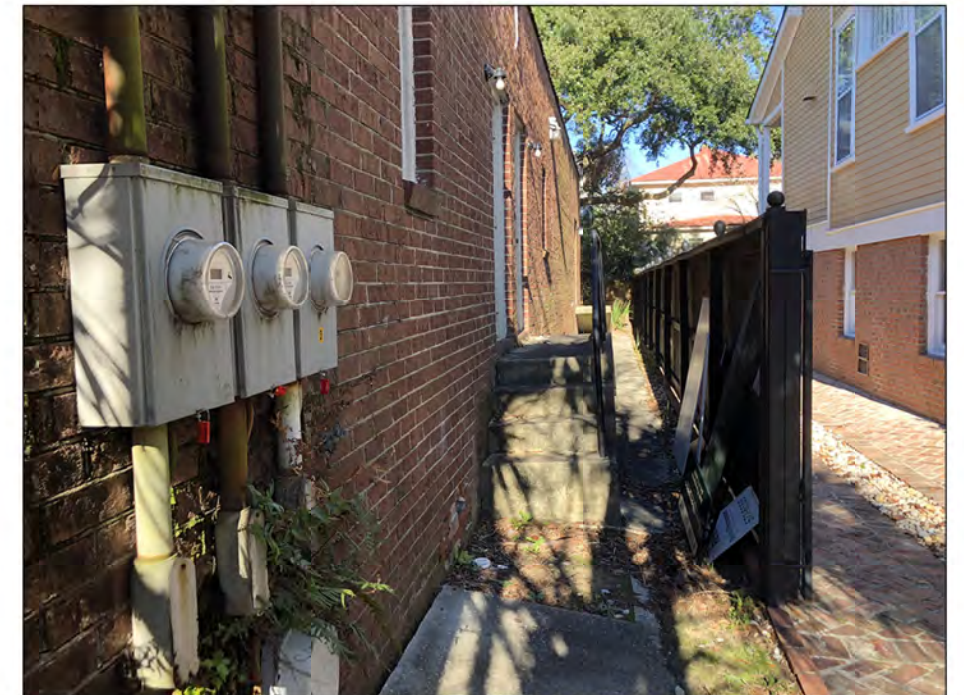
REAR WALKWAY AND STAIRS
