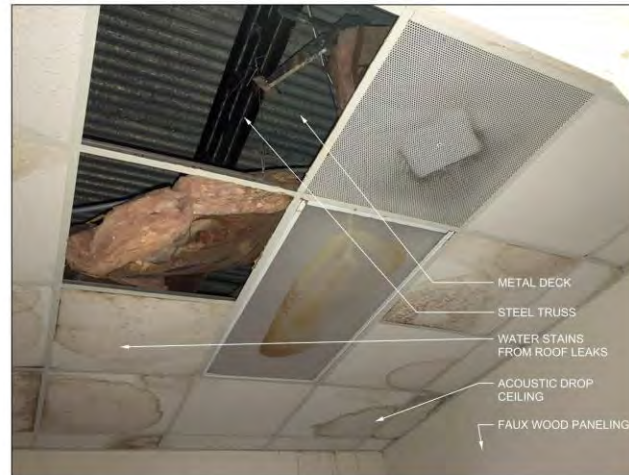
DROP CEILING WITH ROOF STRUCTURE BEYOND
