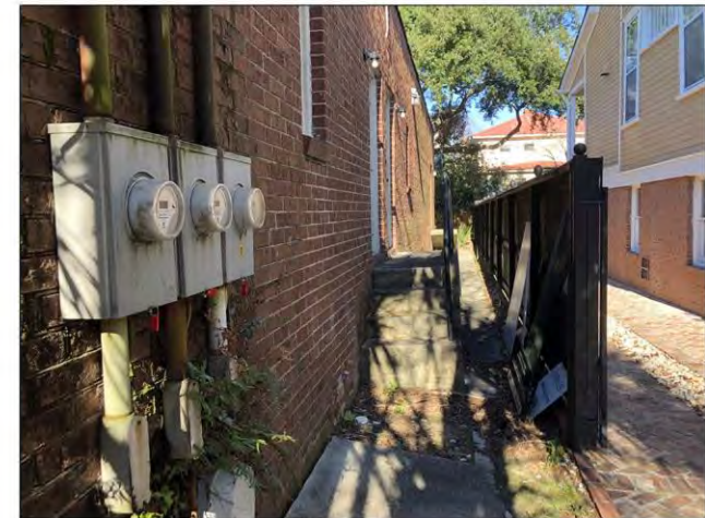
REAR WALKWAY AND STAIRS
