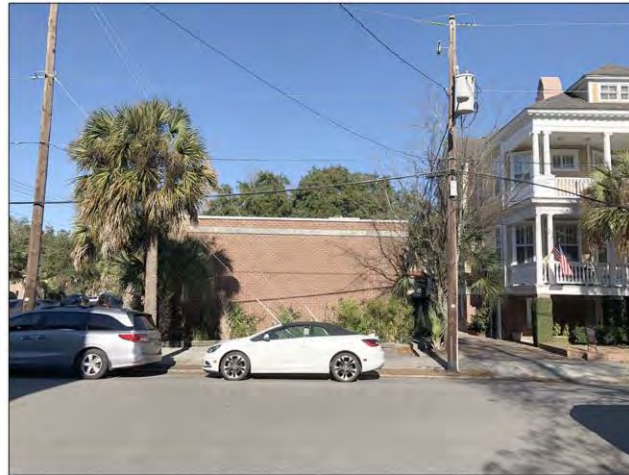
SIDE BENNETT STREET FACADE
