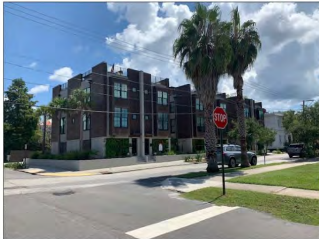
NEIGHBOR ACROSS BENNETT STREET
