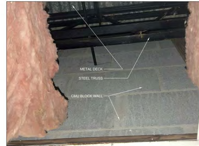
CMU PERIMETER WALL AND ROOF STRUCTURE
