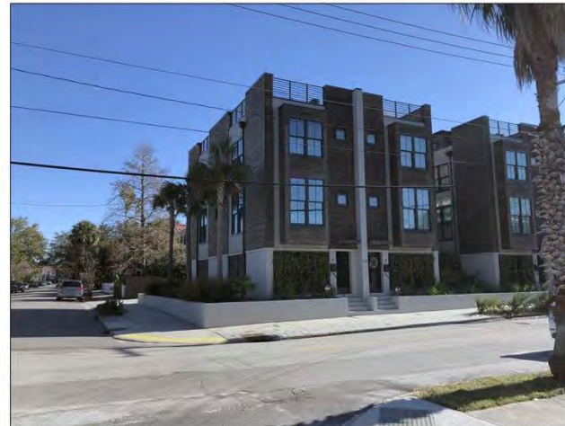
NEIGHBOR ACROSS BENNETT STREET
