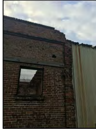
POINSETT DRIVE - BRICK TRANSITION
