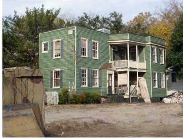
Site Interior - 4 Gadsden St.
