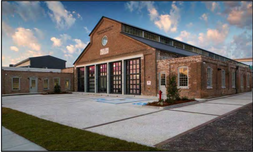
AMERICAN COLLEGE OF THE BUILDING ARTS
