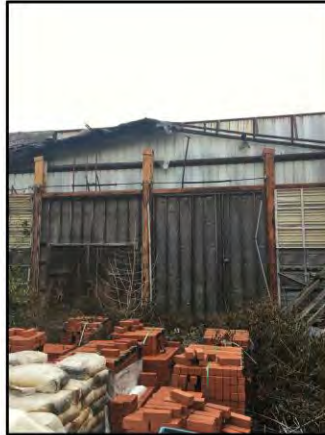
EAST FACADE - INTERIOR
