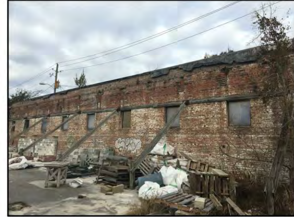
INTERIOR OF NORTH FACADE
